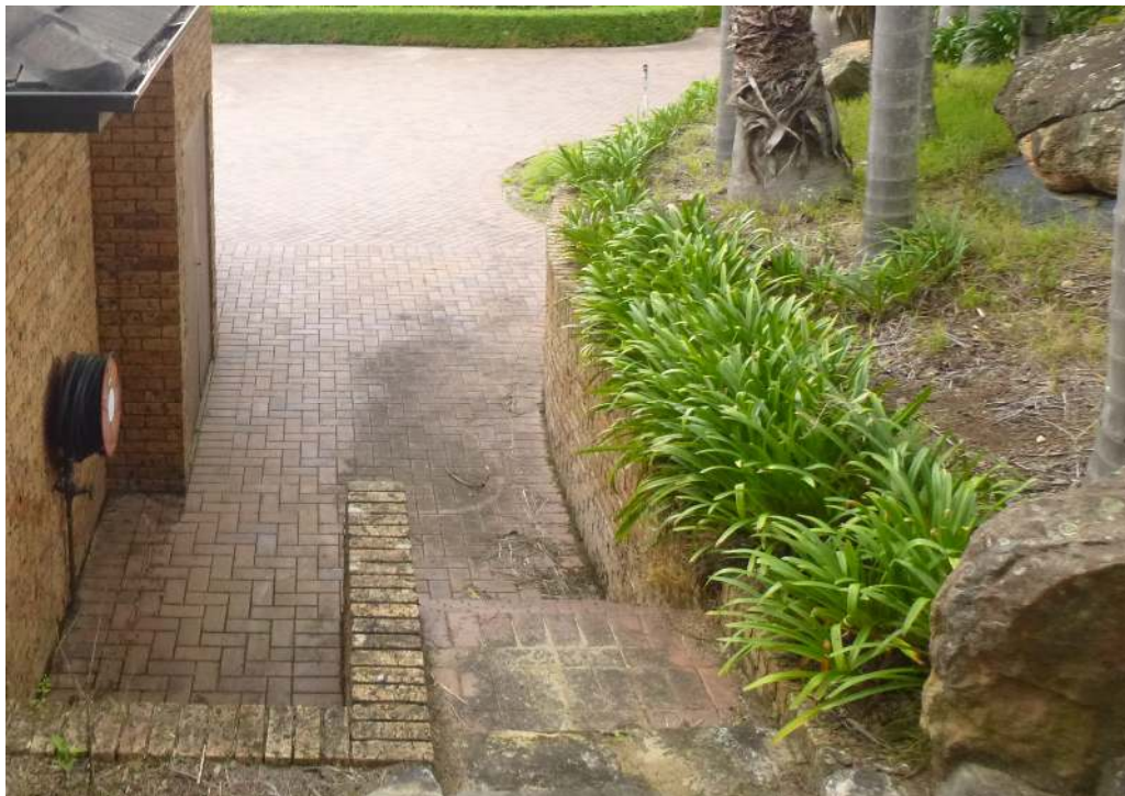
Photograph 16 - Retaining Wall at Residence
