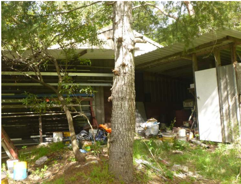
Photograph 7 - Waste Materials at Workshop
