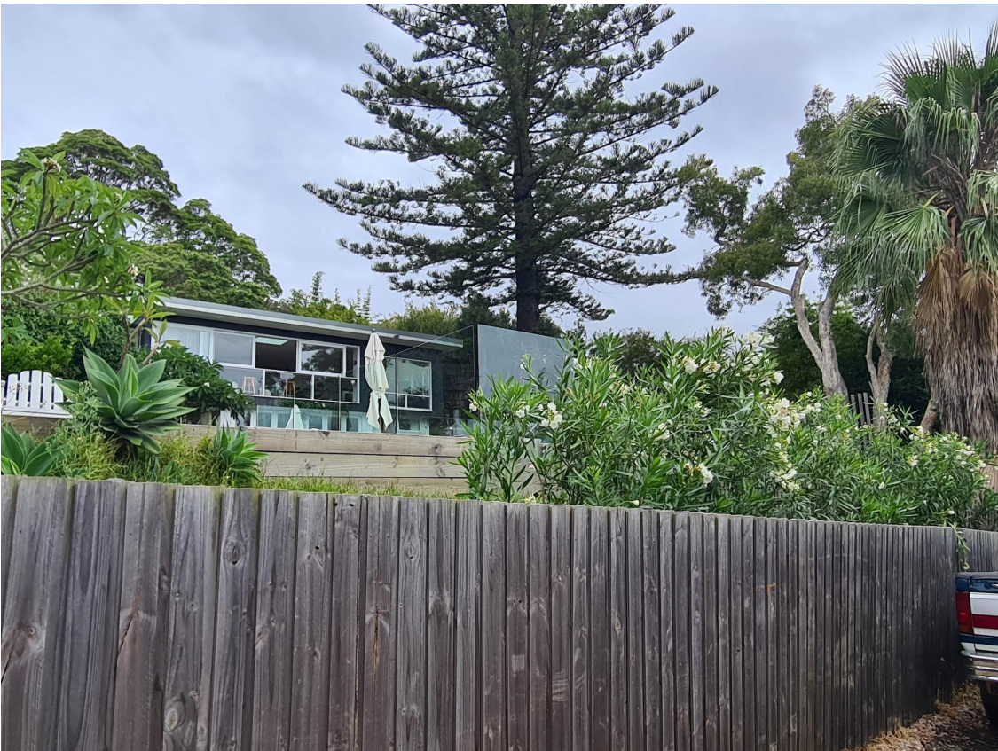
Existing Dwelling at No. 15 Gertrude Ave Newport to the South which shares a boundary with the shared driveway access
