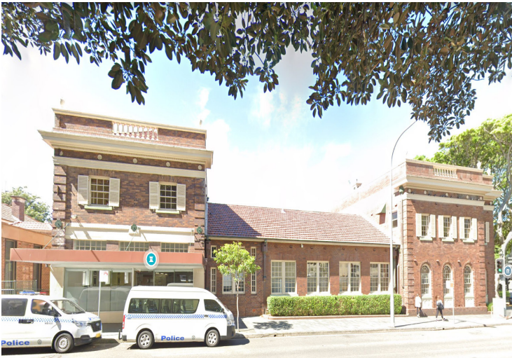
Manly Court House and Police Station
