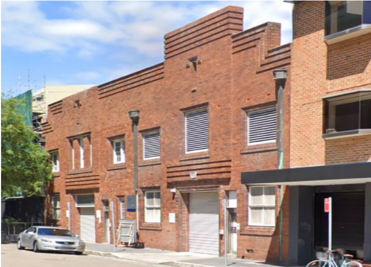
Electricity Substation, 34A-36 Whistler Street
