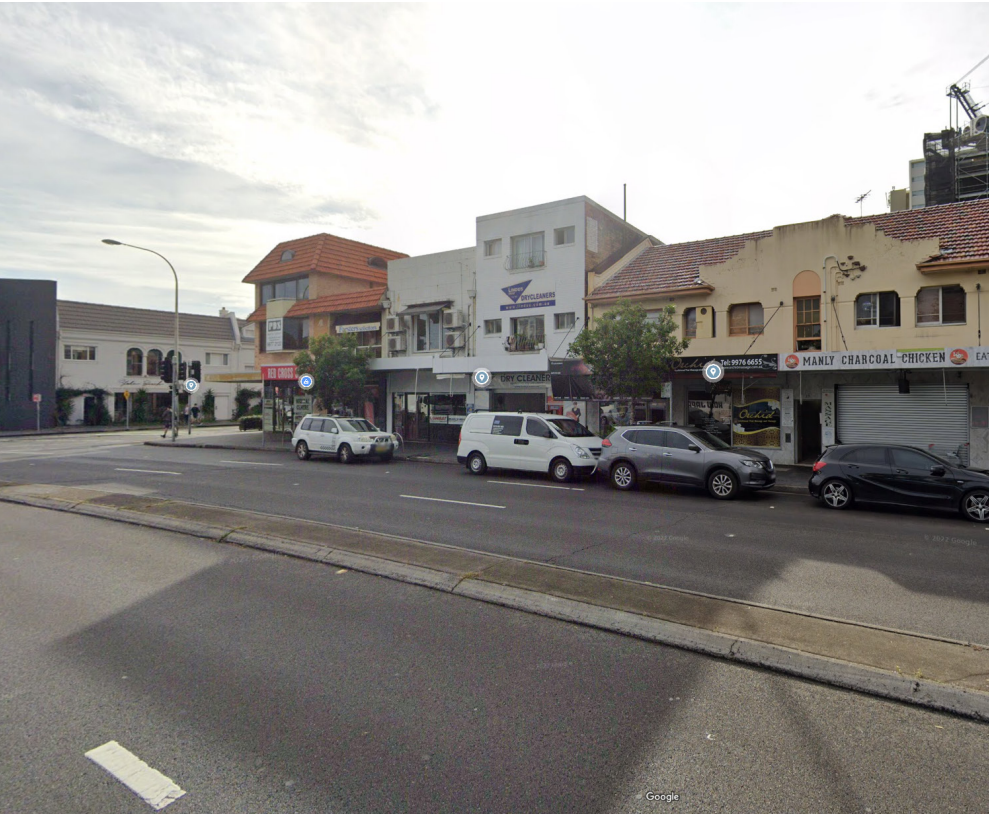
Belgrave Street looking north-east towards the site
