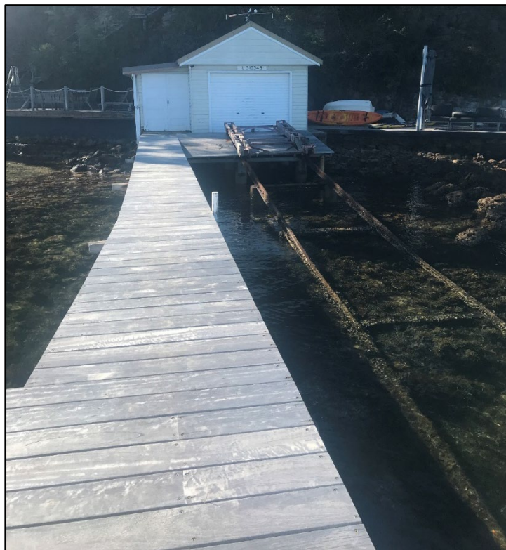
Figure 7 - Northern neighbours facility looking towards shore (photo taken in 2020)
