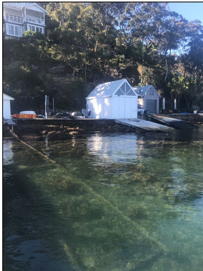
Figure 3 – Existing boatshed, timber decking and metal skid ramps (photo 2020)
