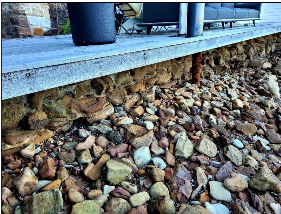
Figure 5 – Existing seawall with timber decking over top (photo taken 19/5/22)
