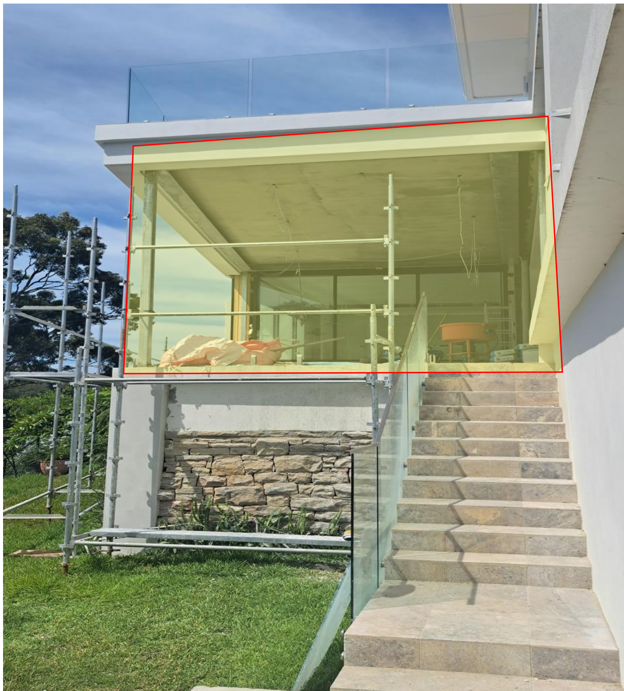
Figure 15: The covered terrace area highlighted in yellow, which is built above the approved footings (source: Gyde)
