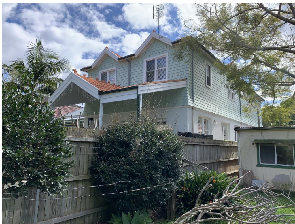
Fig 11: View looking north-west towards the rear elevation of the adjacent dwelling at No 50 Johnson Street
