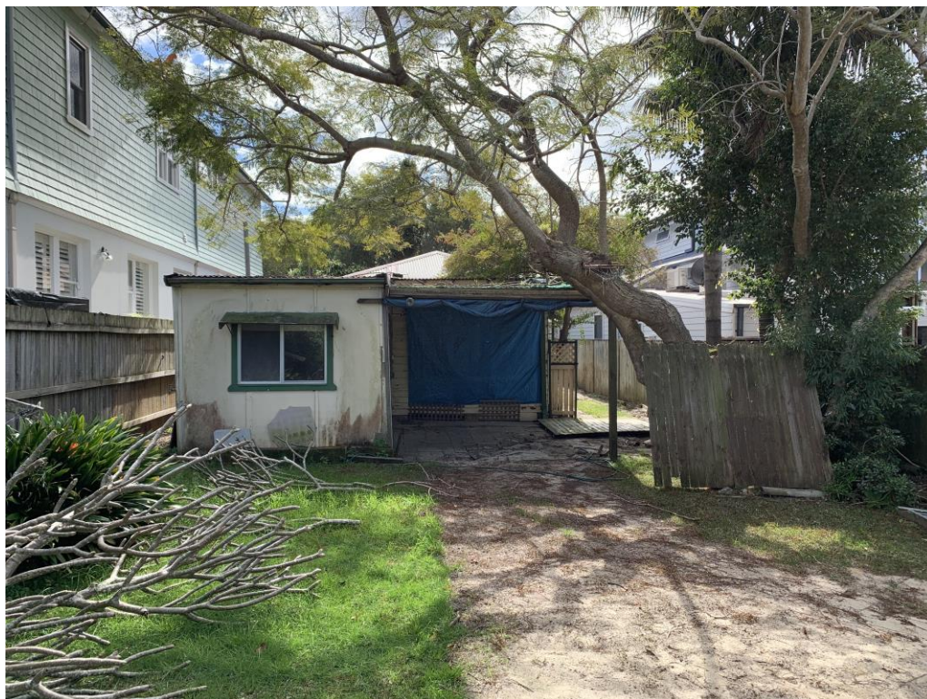
Fig 10: View of the rear yard and rear elevation of the subject dwelling, looking north
