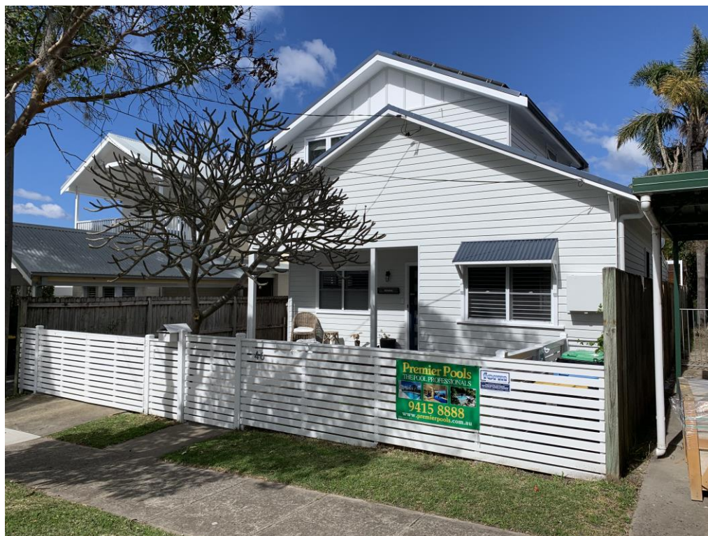
Fig 5: View of adjacent dwelling at No 46 Johnson Street, looking south-east
