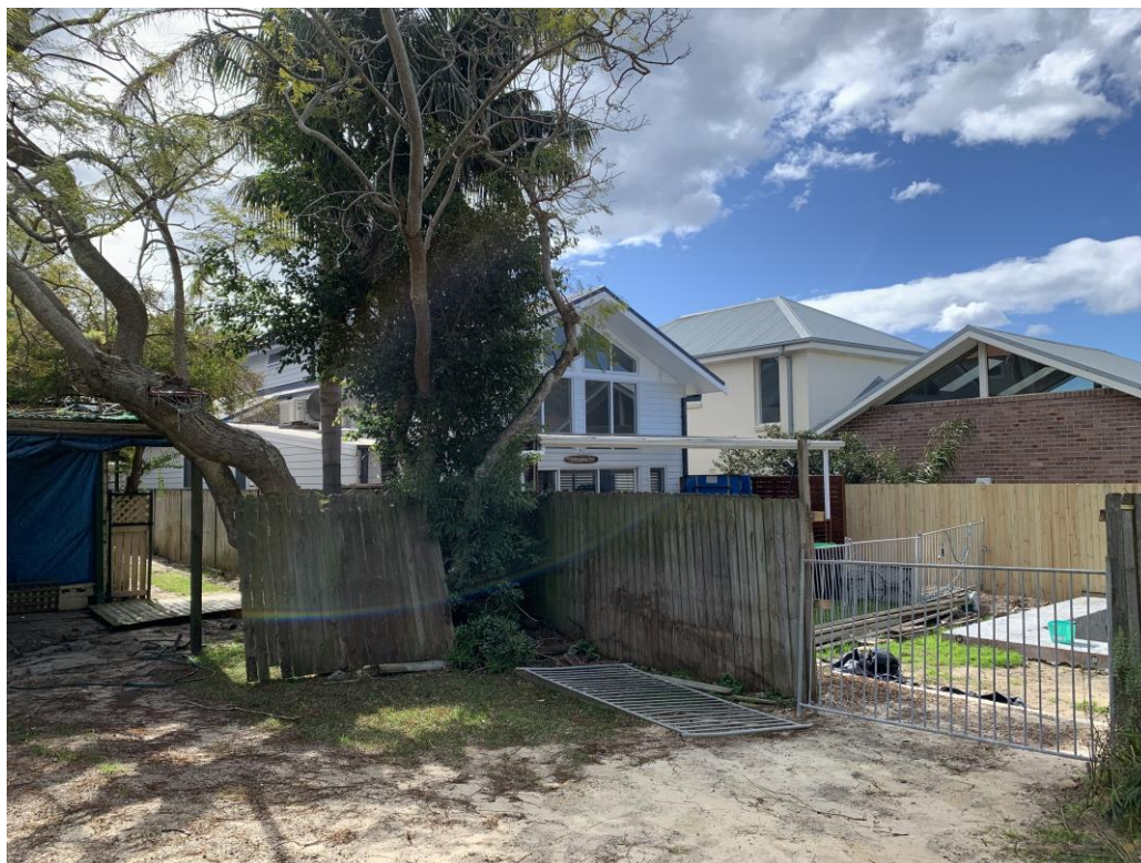
Fig 12: View looking north-east towards the rear elevation of the adjacent dwelling at No 46 Johnson Street
