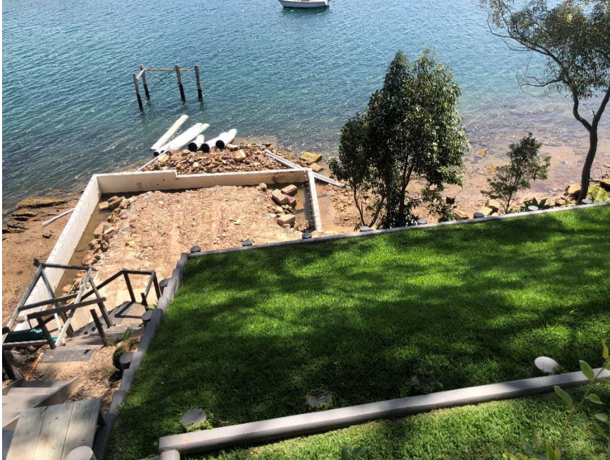
Photo 1 Dintel foundation wall enclosing demolished former boatshed. Toe of former ramp just visible below the waterline beyond the pile of demolished materials
