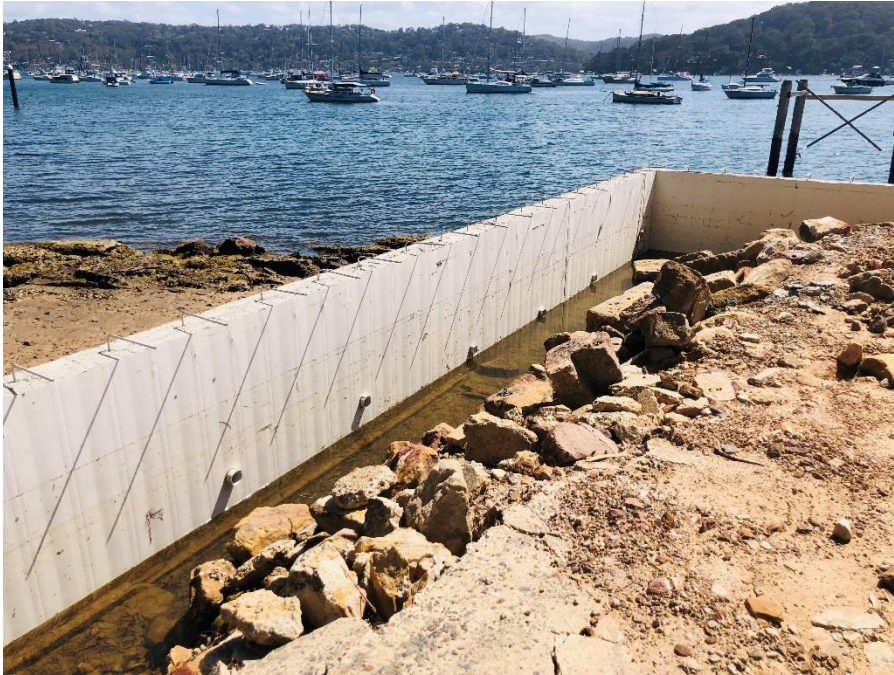
Photo 3 Southern Dincel foundation wall with outer poles of former jetty behind
