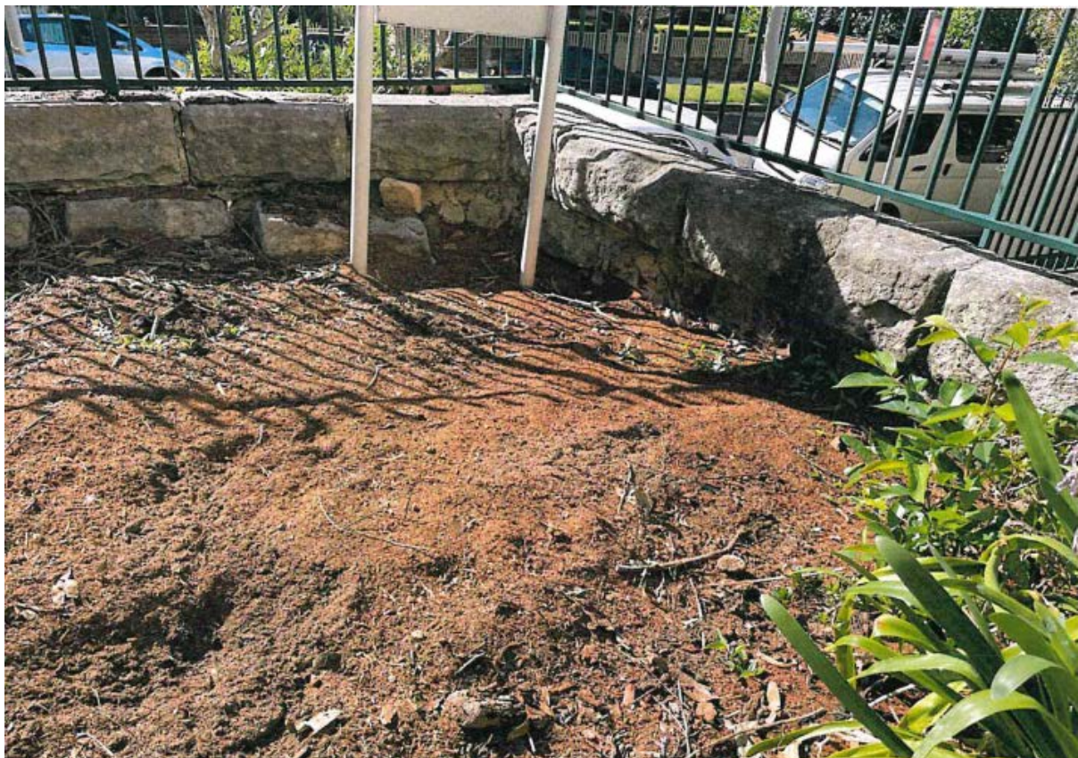
Photo 4 – View of Works Area A from Birkley Road (following tree removal).
