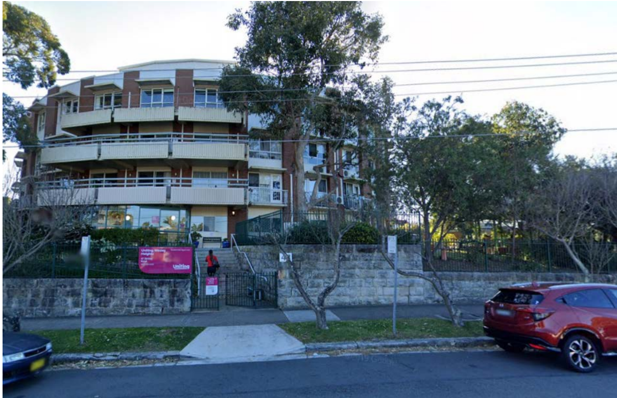
Photo 1 – View of Works Area A from Birkley Road (showing tree now removed behind wall)
