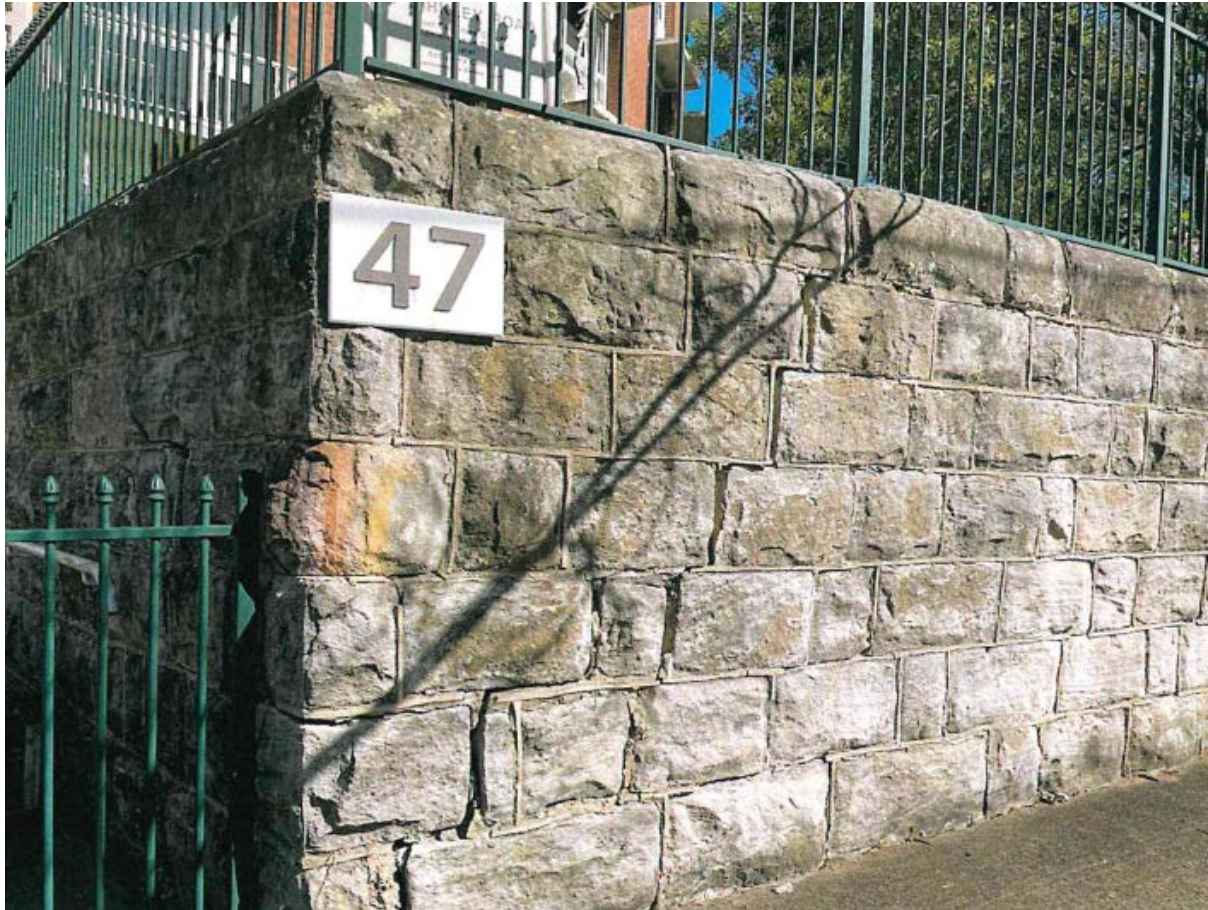
Photo 3 – View of Works Area A from Birkley Road (following tree removal).
