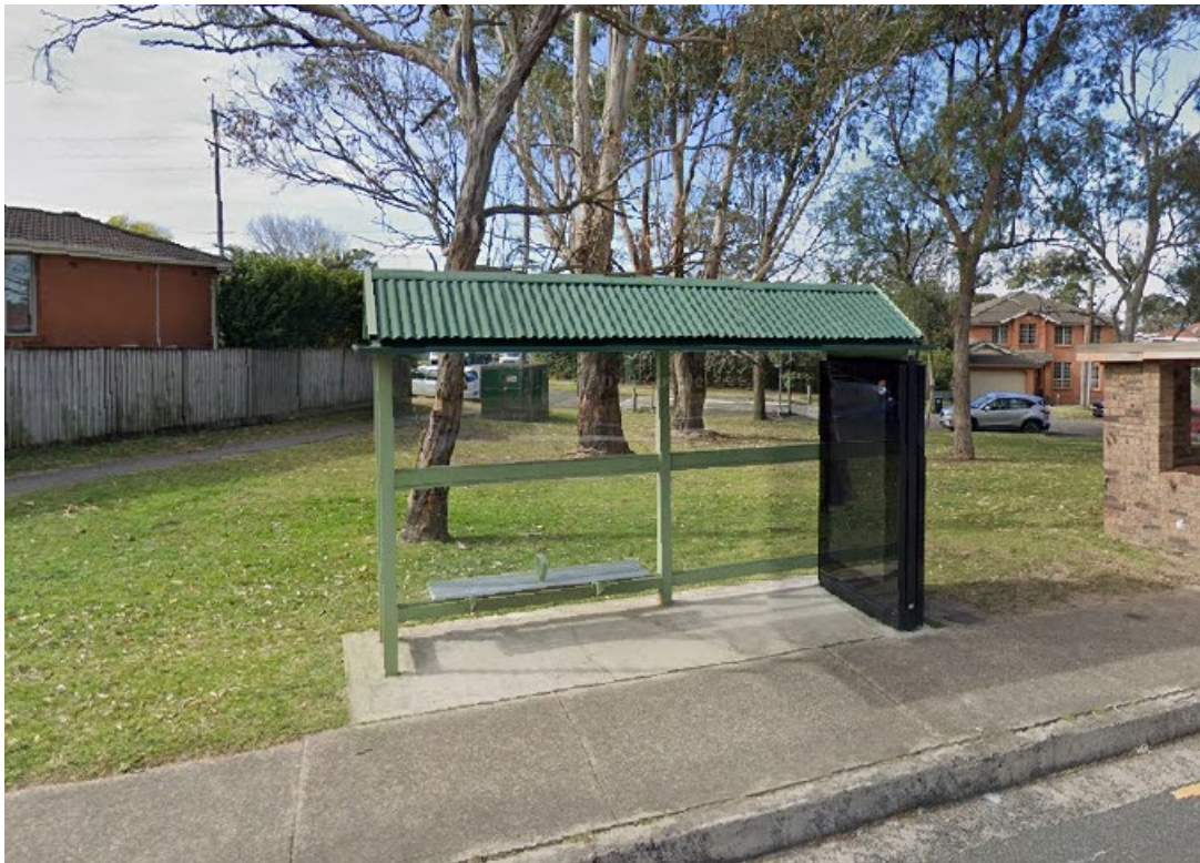
Figure 5: View of G2 Shelter and Advertising Signage Panel
