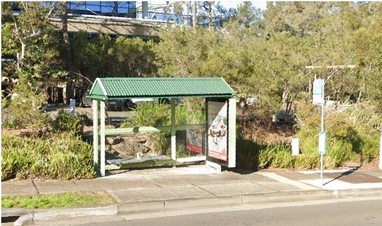
Figure 3: View of G1 Shelter and Advertising Signage Panel
