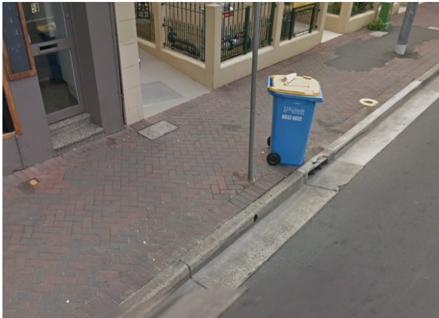
Figure 3 - Existing Kerb and Channel Outlets (Google Street View accessed 27.08.19)
