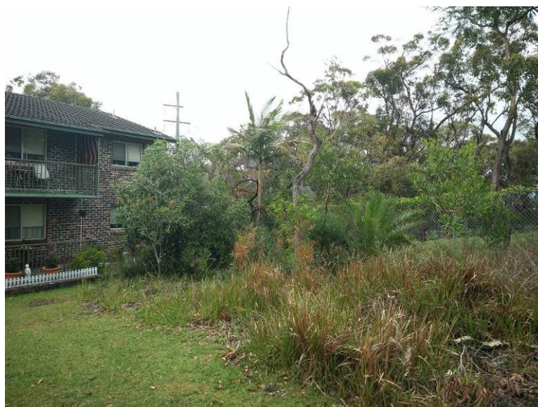
Photo 8 & 9 – Vegetation requiring further maintenance
