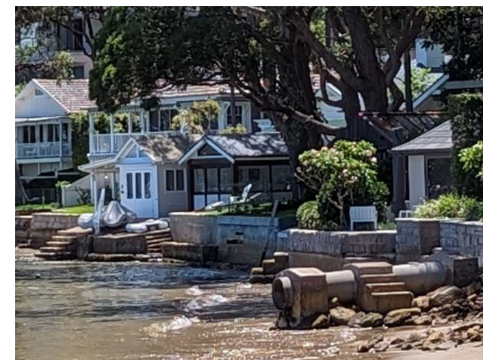
GLAZED DOORS TO WATER SIDE
