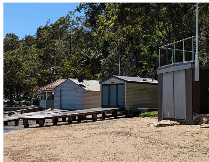
GLAZED DOORS TO WATER SIDE
