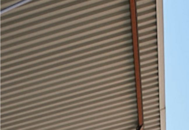
CORRUGATED COLOURBOND ROOF (SR)
