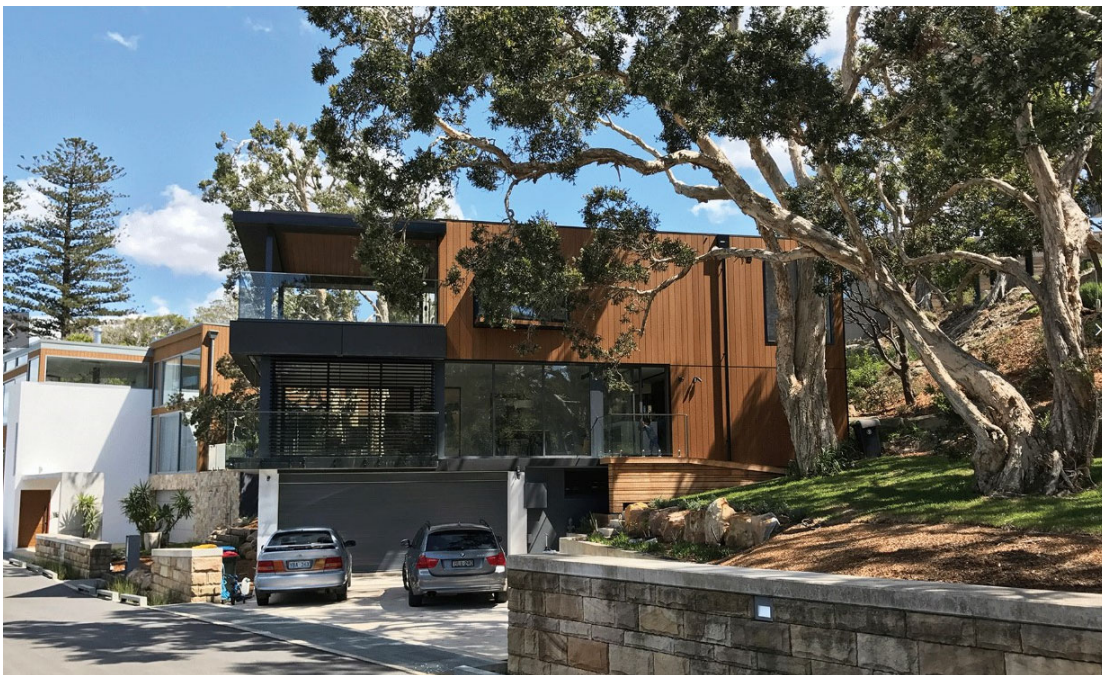
Image 5. Street view – East of the development site showing existing mature landscape and embankment to rear of site. Image source: Innwood
