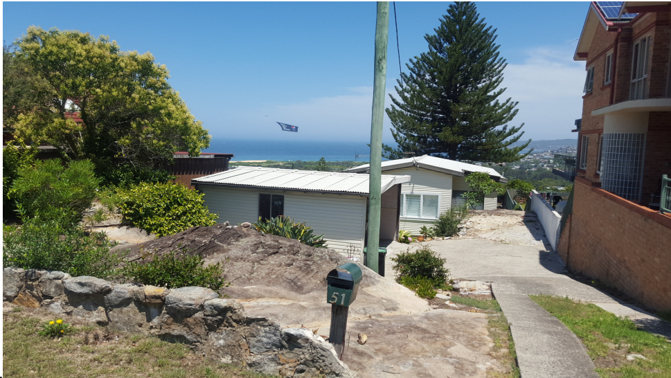
51 Quirk St. View of the existing house from the front footpath
