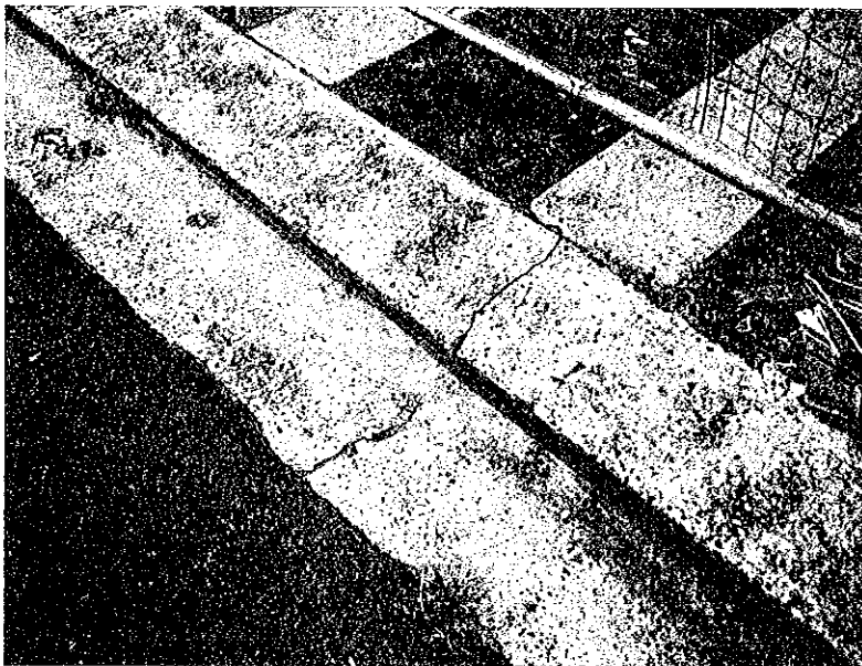
Cracks of Dish Drain and grate in middle of site
