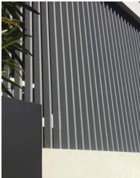
PRIVACY SCREEN Vertical metal privacy screen with max. 30% transparency to achieve BAL-40. Decowood or similar. Colour: TBA
