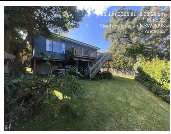
Photo 2: Southwestern corner and southern face of the residence
