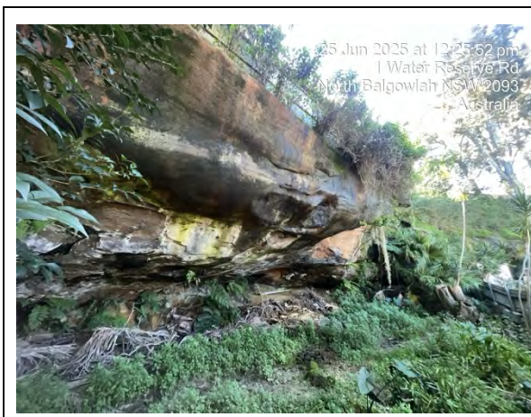
Photo 3: Looking north-east along undercut sandstone escarpment in the rear of the site.
