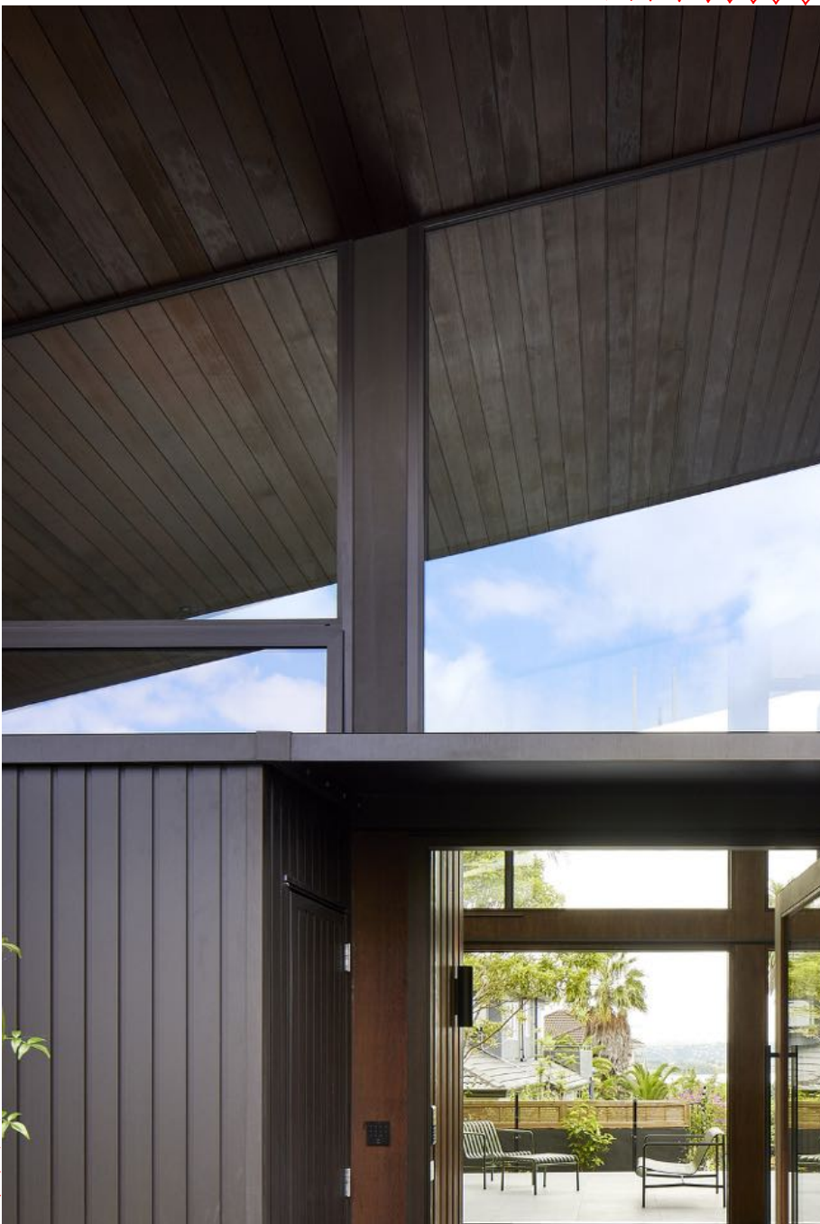
AM + GL1 _ ANODISED ALUMINIUM WINDOWS + CLEAR GLASS
