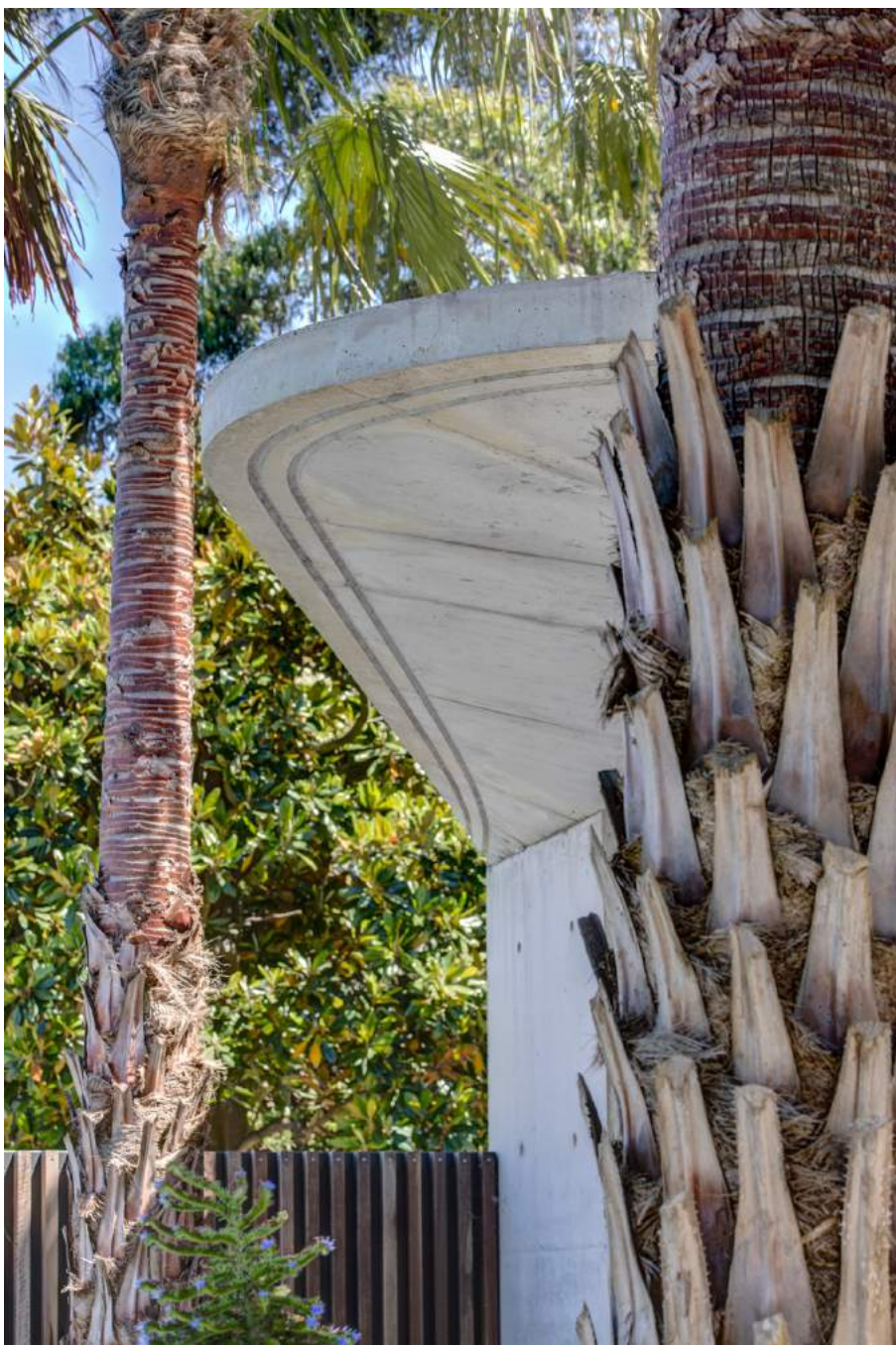
CONC2 _ NEW OFF-FORM CONCRETE
