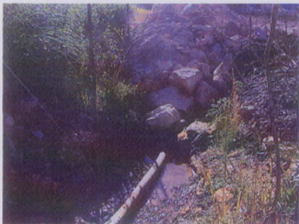
Plate 3. Channel to be battered back and replanted
