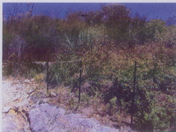
Plate 14. Stormwater drainage ditch showing weed plume and slope where water drains onto the site.
