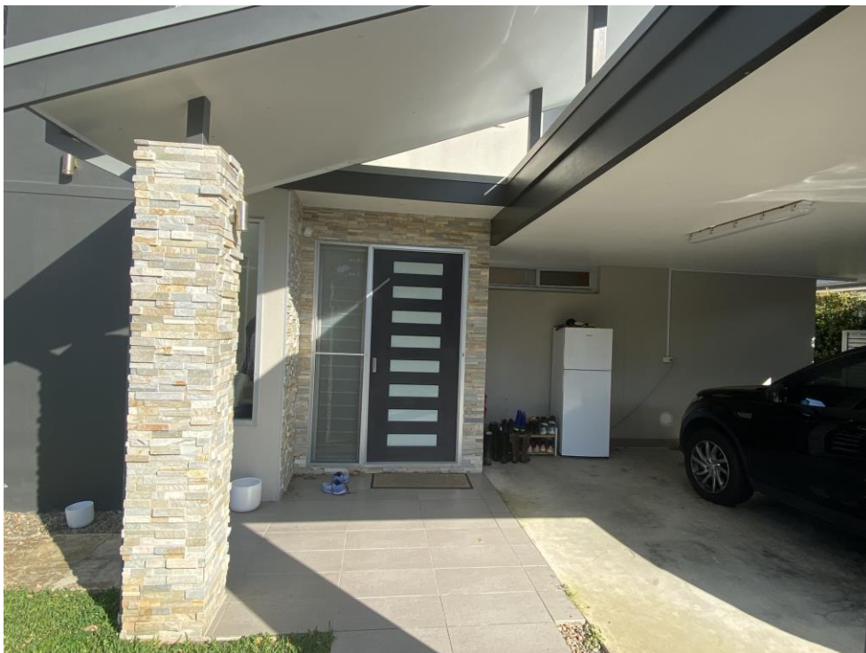
Figure 5. The existing front entry to the dwelling that is to be modified under this application
