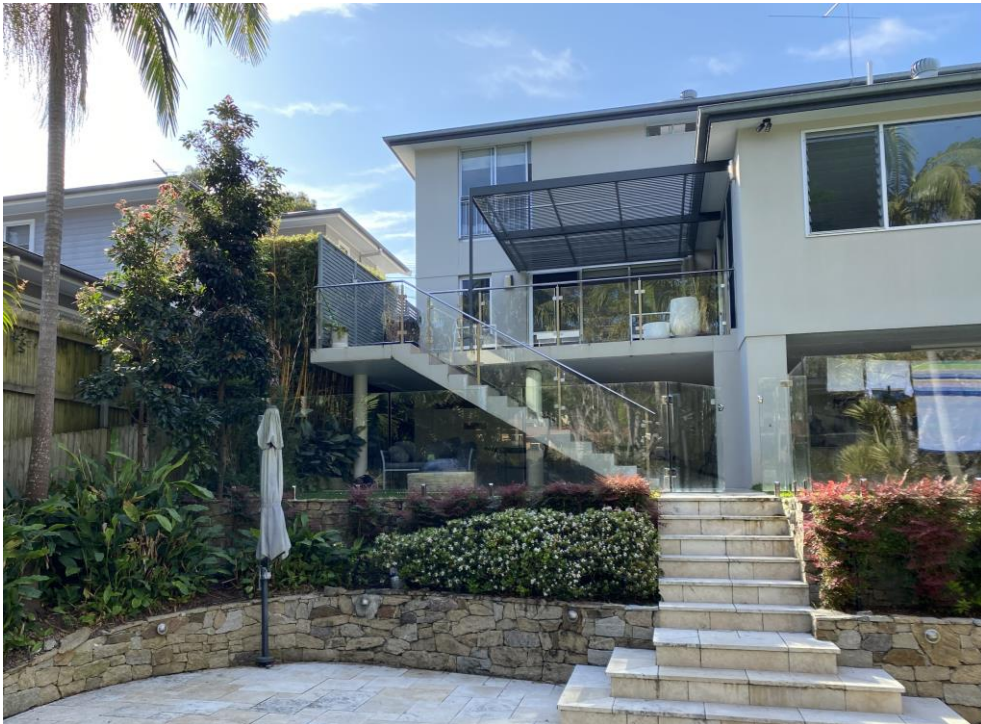
Figure 7. Looking east towards the rear ground floor level and proposed location of the modified roof form over the alfresco area
