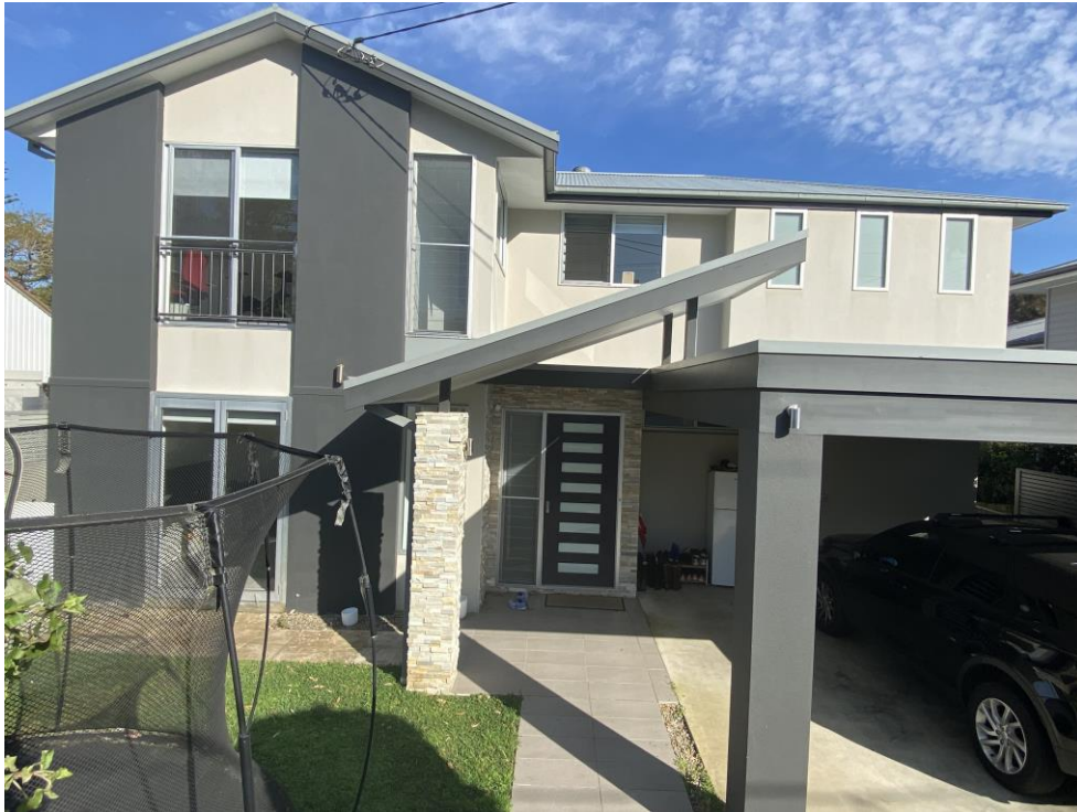
Figure 4. Looking west towards the front of the existing dwelling
