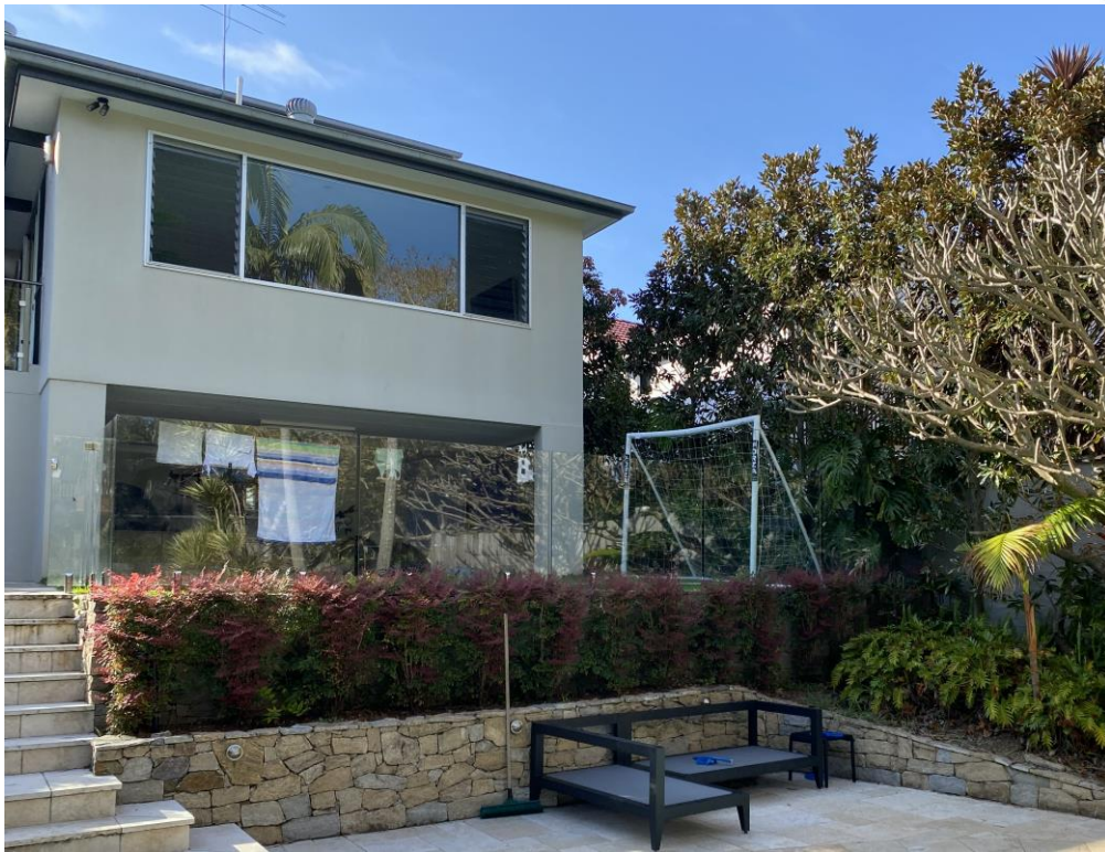
Figure 8. Looking south-east towards the rear of the living area, the roof form to be retained as existing.
