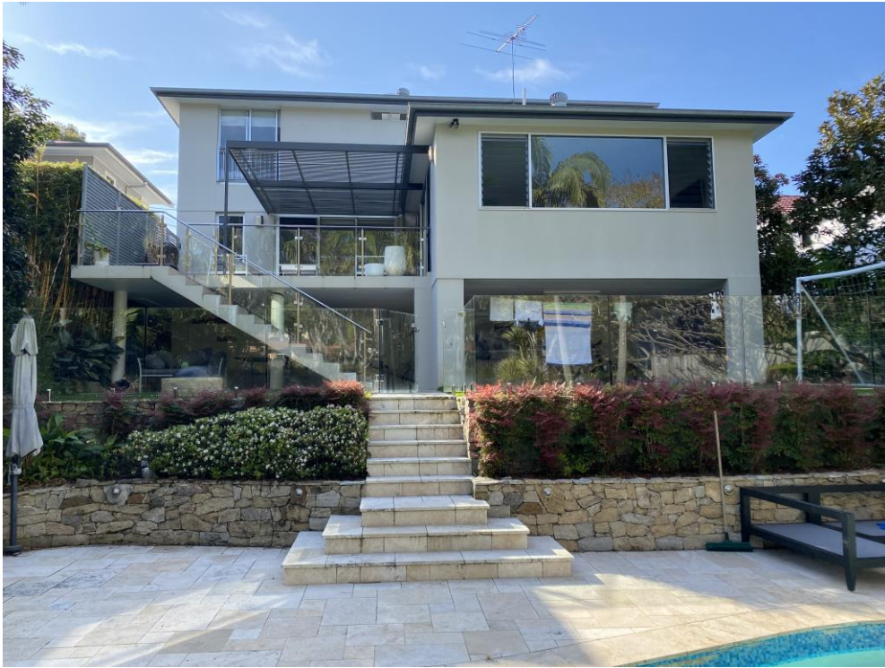
Figure 6. Looking east, the existing rear elevation of the dwelling
