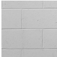
1. Existing Concrete Block Wall Colour: White
