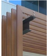
9. Timber Looking Lift Lobby Screening
