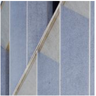
5. Precast Concrete Panels
