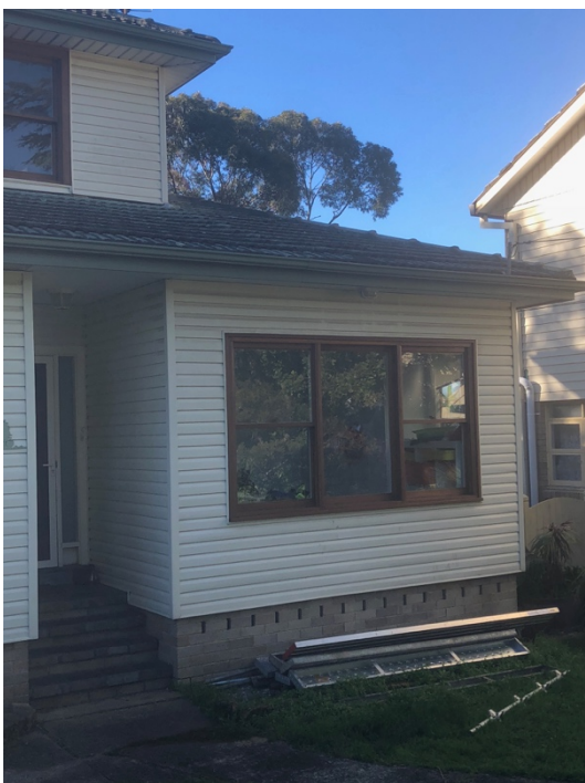
FIGURE 4 FRONT (SOUTH) ELEVATION
