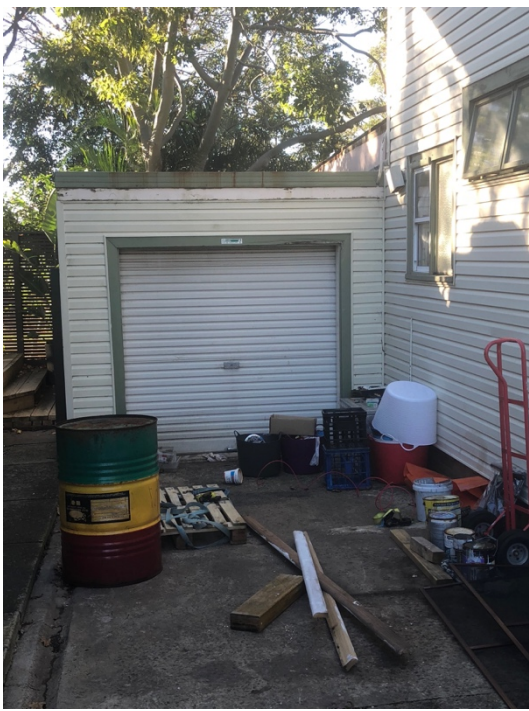
FIGURE 2 VIEW OF DRIVEWAY
