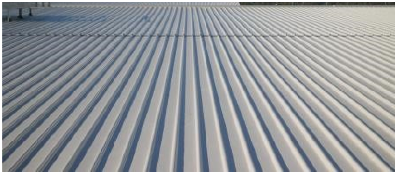
COLOURBOND "DUNE" MINI ORB ROOFING TO MATCH EXISTING
