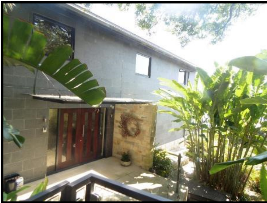
South elevation of whole dwelling
