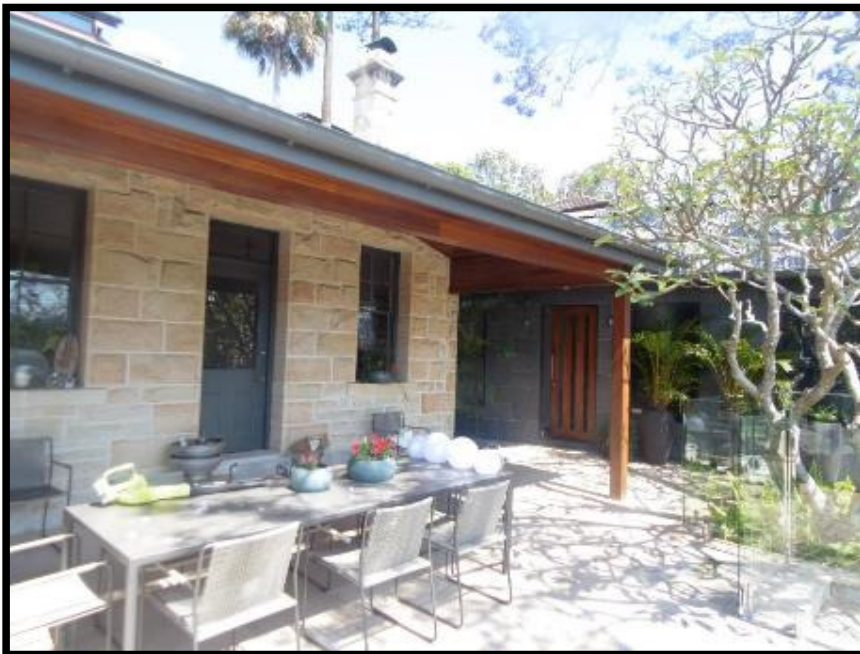
Heritage listed east facing sandstone wall
