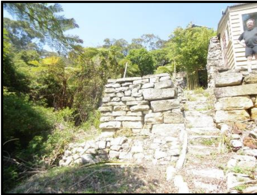
Existing drystone wall
