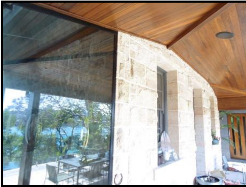
New window to heritage listed east facing sandstone wall
