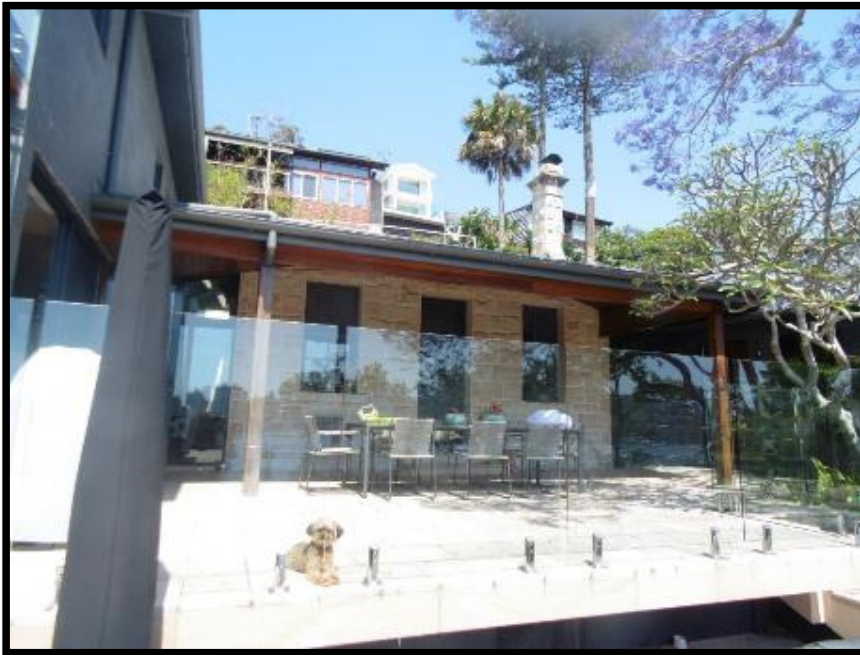
Heritage listed east facing sandstone wall
