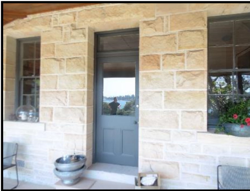
Door to heritage listed east facing sandstone wall
