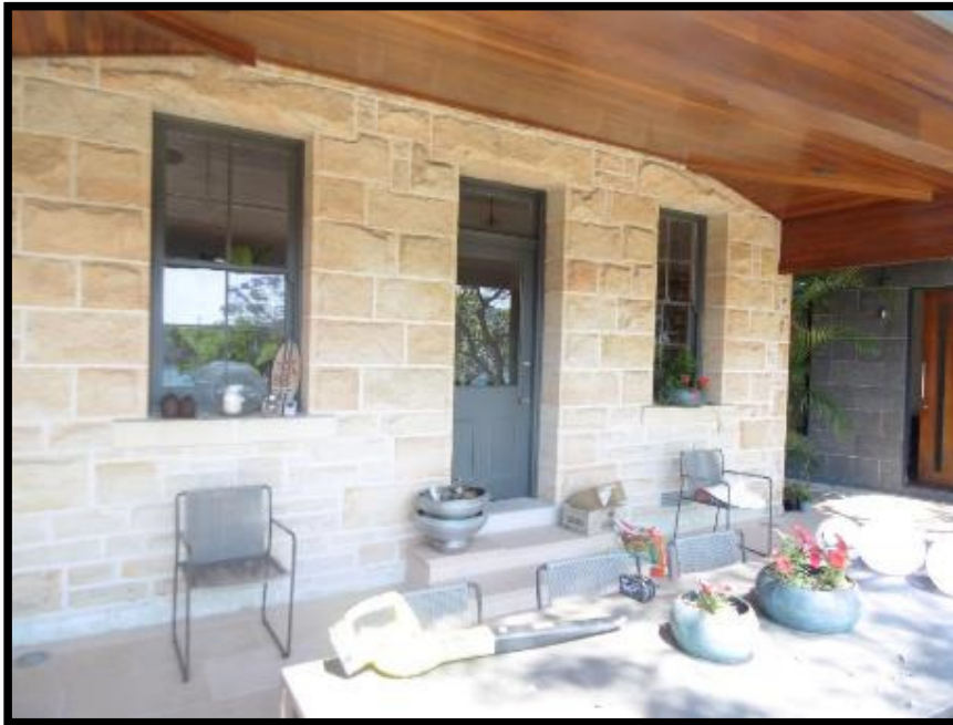
Heritage listed east facing sandstone wall
