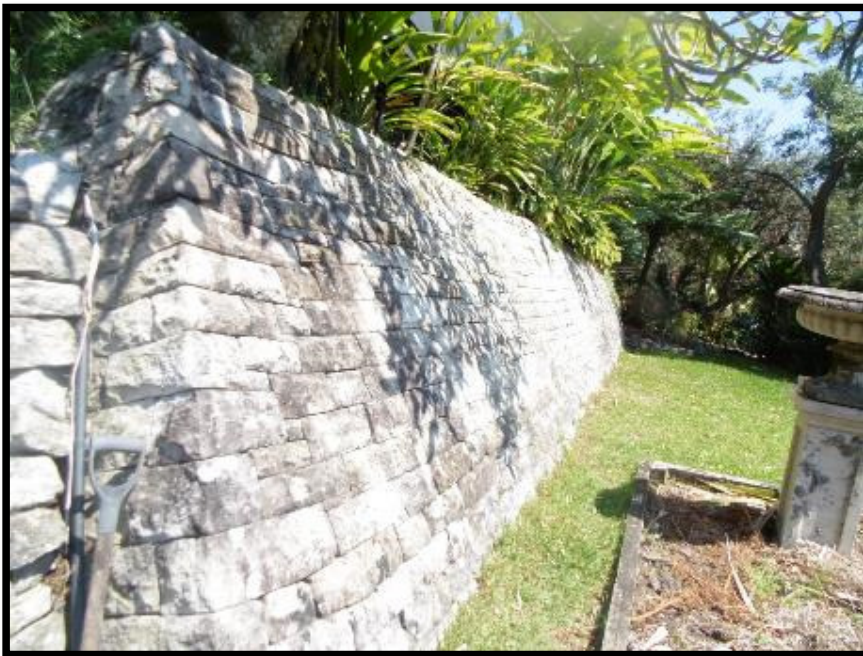
Existing retaining walls to the site
