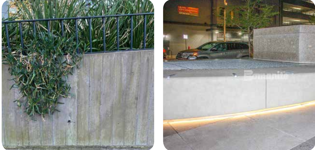
Beton brut concrete wall Wall strip lighting
