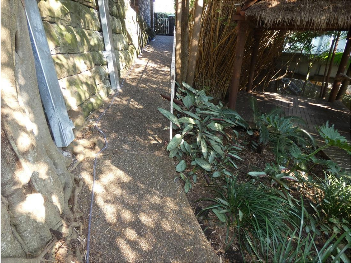
Photo 3: The sandstone retaining wall bordering Bower St and pathway leading to the front garden. Note the gazebo on the right and adjoining clump of bamboo.
