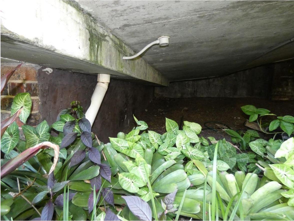
Photo 7: The underside of the concrete driveway was assessed as potential roosting habitat for microbats.
