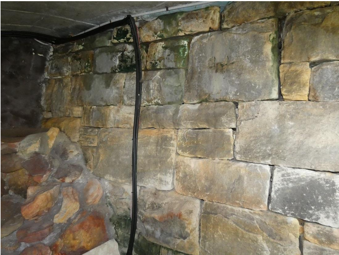
Photo 8: The cavities in the sandstone retaining wall underneath the driveway and away from the driveway was assessed as potential roosting habitat for microbats.
