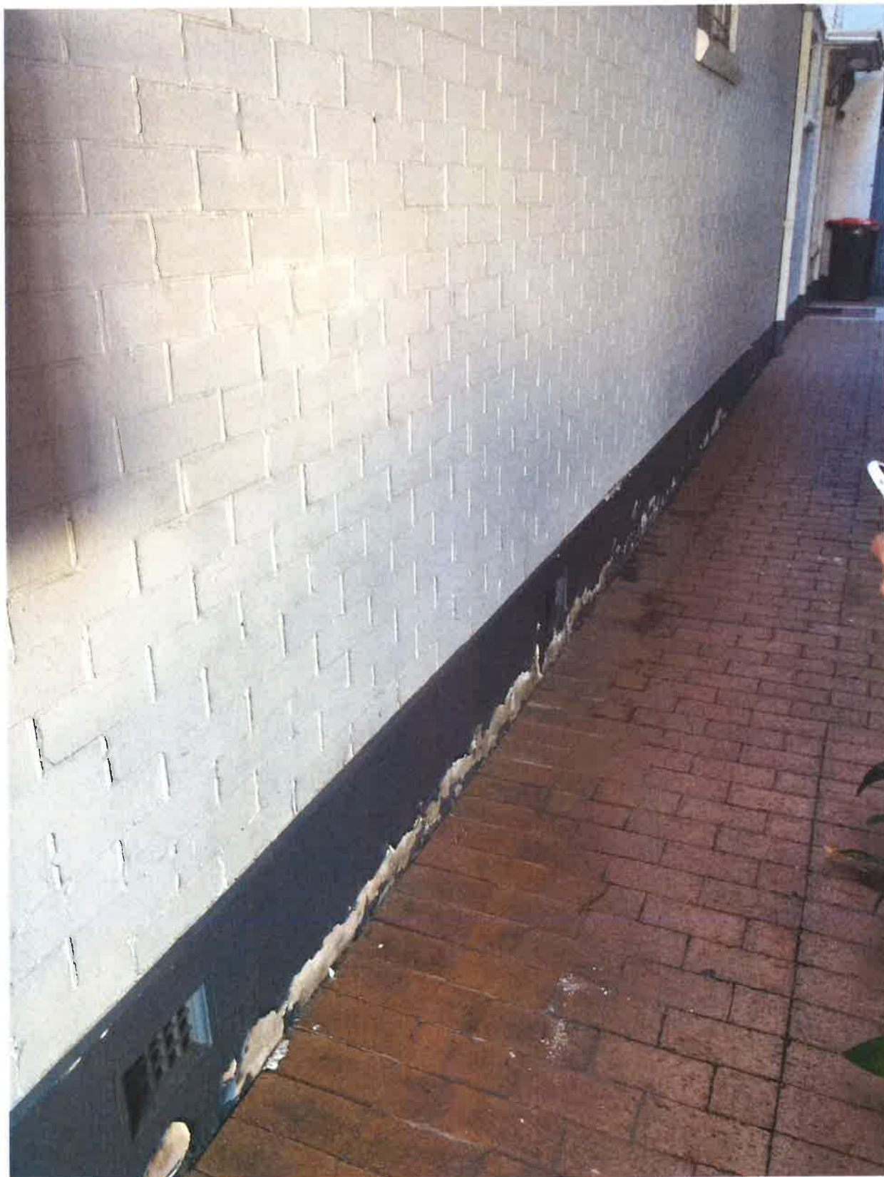
P07 – Tucking pointing to brickwork and rising damp above the footing.
