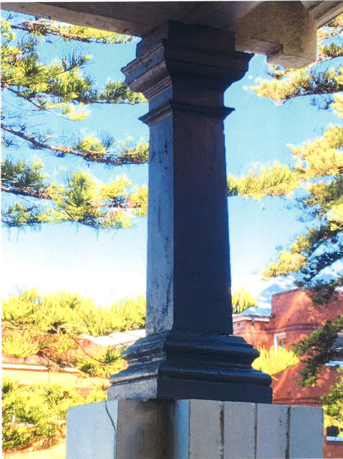
P18 - Timber post supporting the balcony roof exhibiting rot and is distorted.
