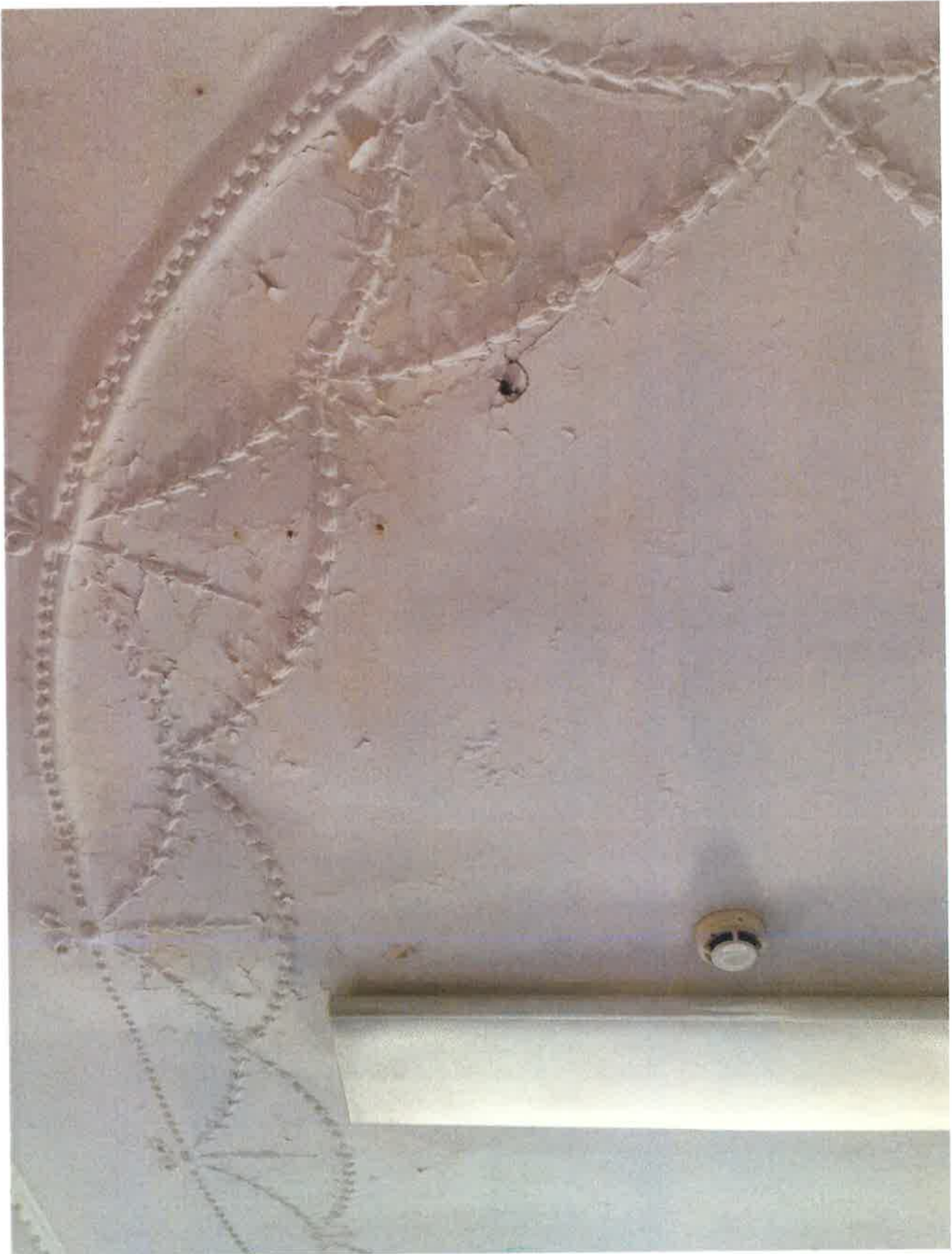
P08 – Damage and sagging to the ceiling to the front first floor room.
