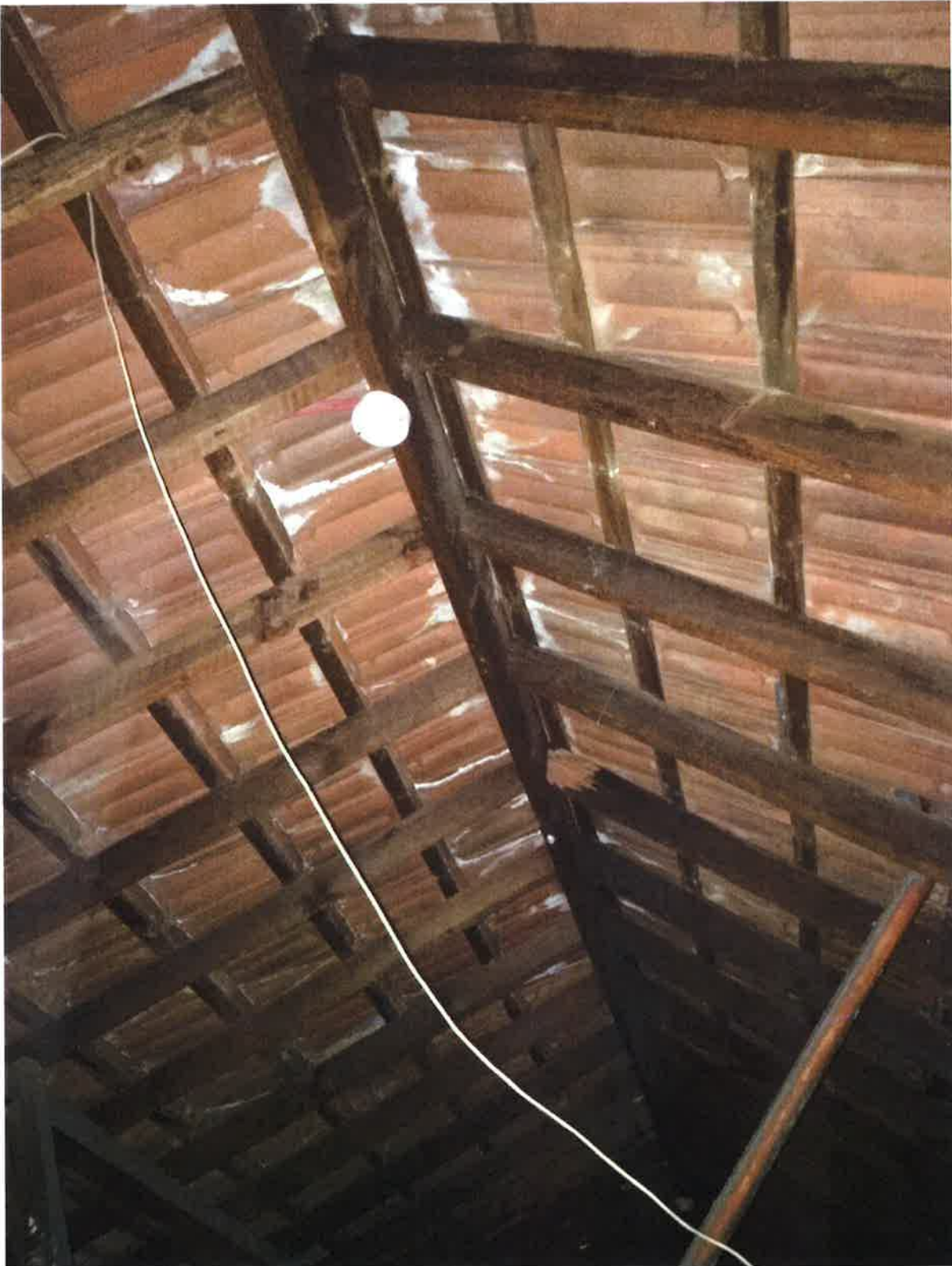
P20 - Efflorescence to underside of roof tiles.
