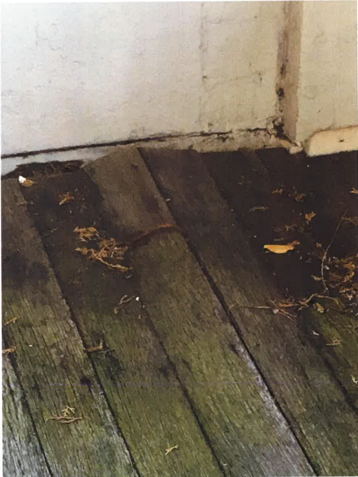
P12 – Buckling to first floor balcony floor boards.
