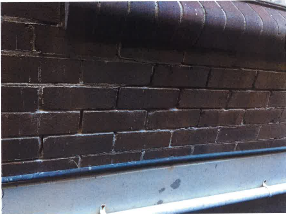
P10 – Fretting to façade brickwork.
