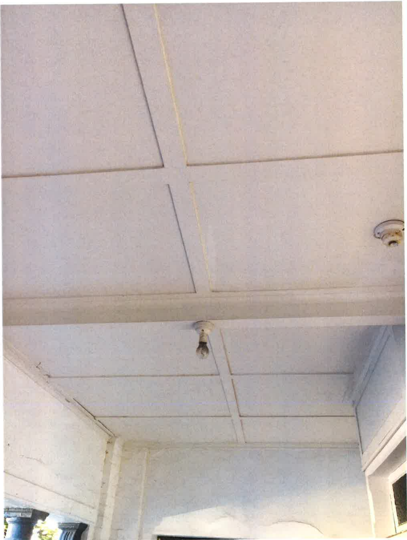
P05 – Asbestos ceiling lining to front entry.
