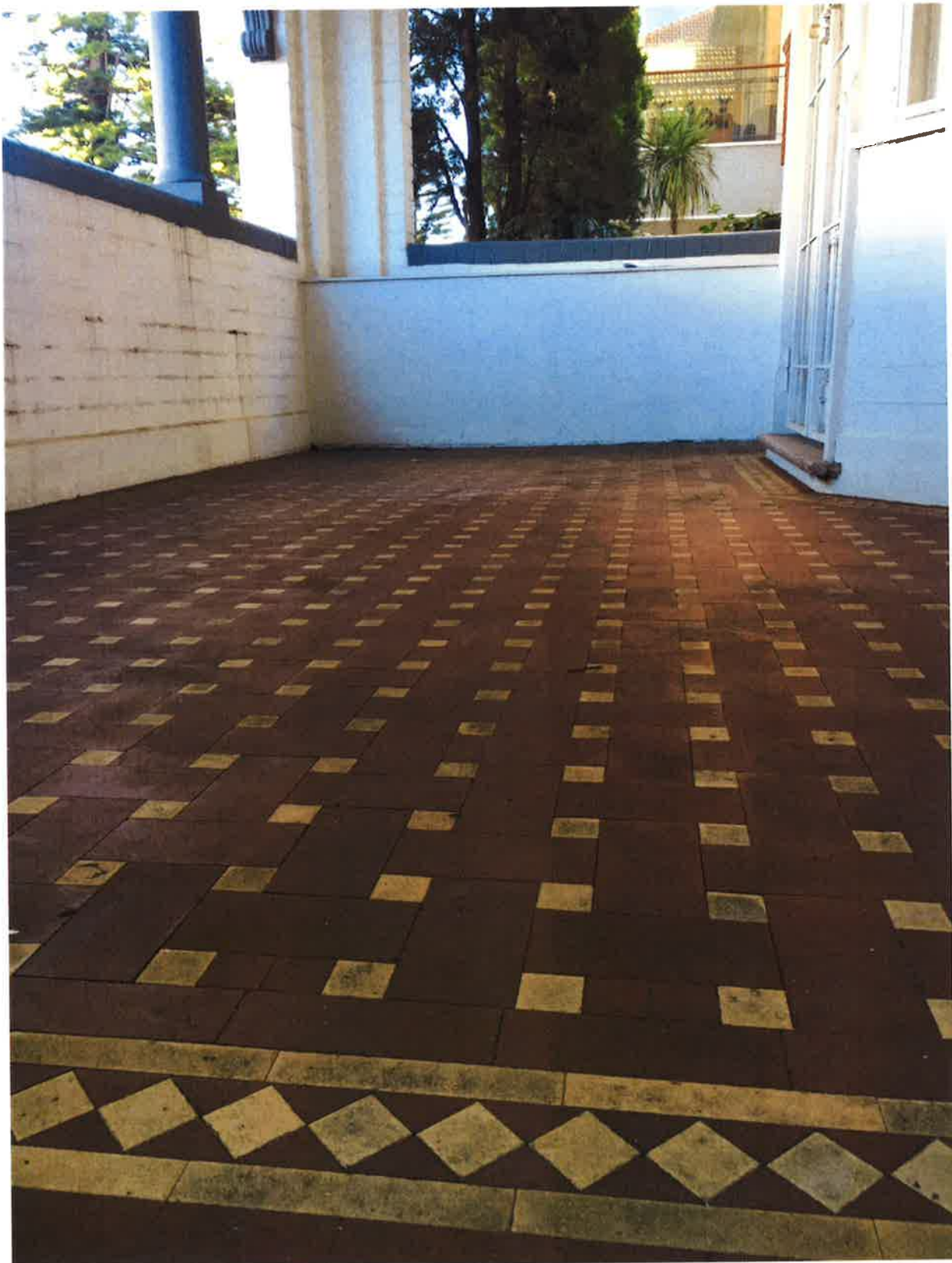
P06 – Front entry porch slab out of level.
