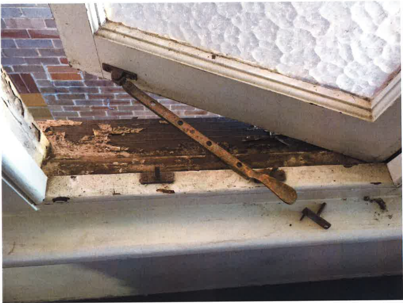
P16 – Weathering and rot to the north-eastern external window frames.
