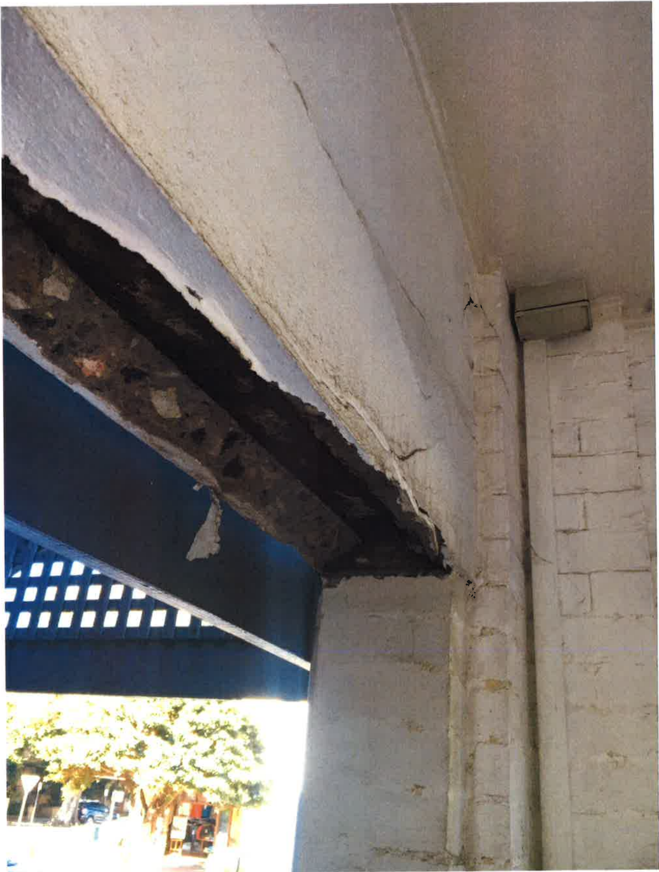
P03 – Spalling to beams and corroded lintel bars.
