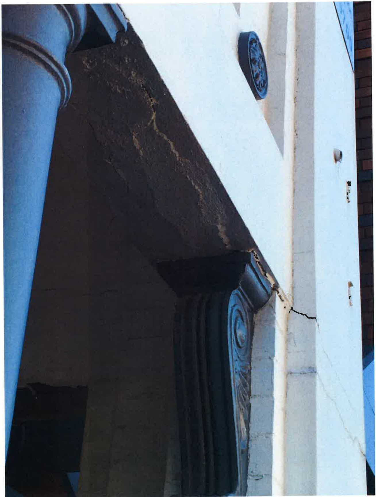
P02 – Separation to brickwork at corbels.
