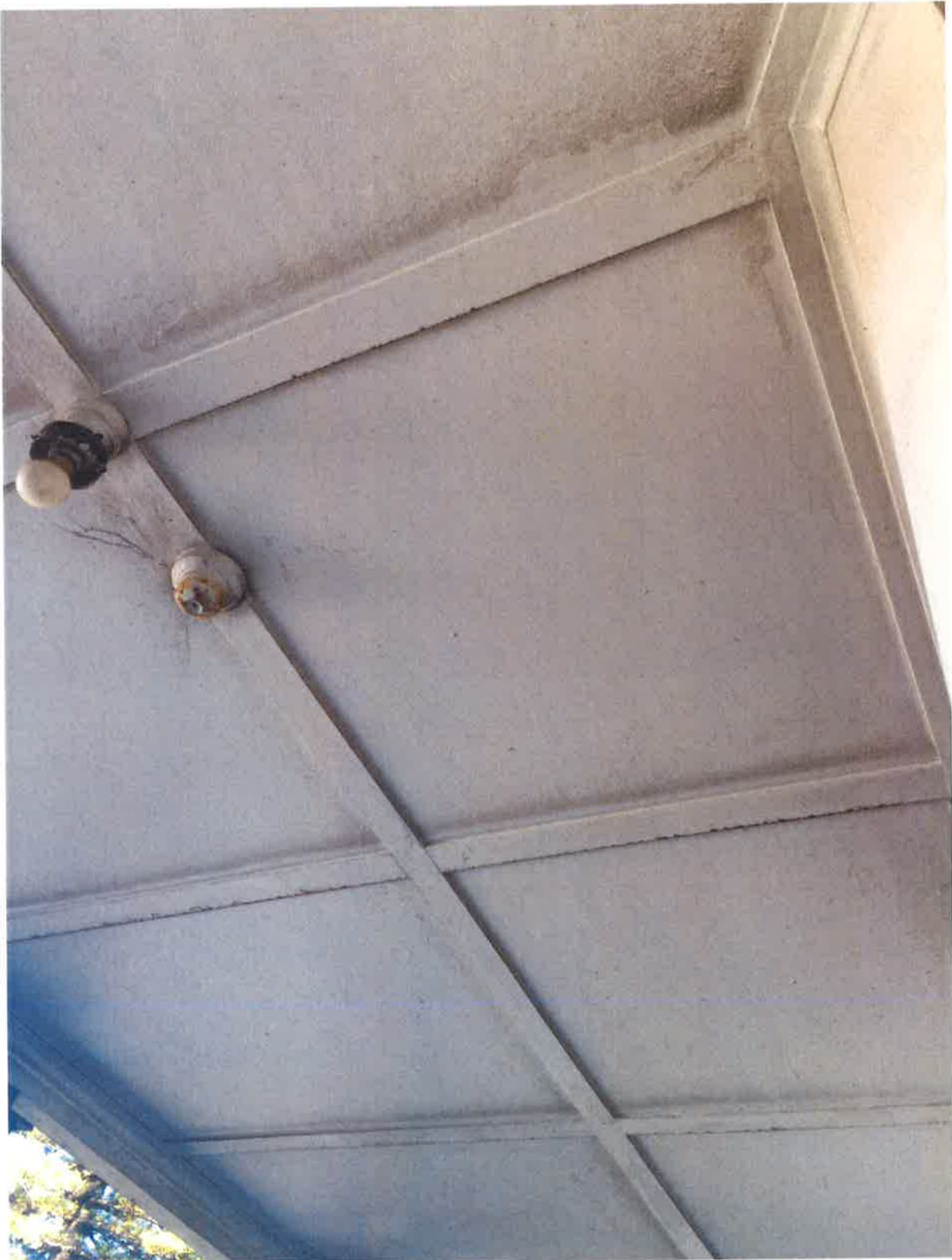
P09 – Asbestos ceiling lining to front first floor balcony.
