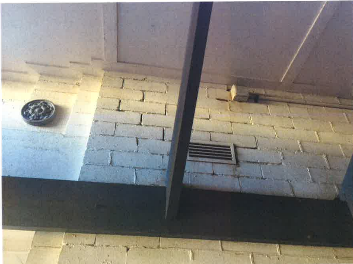
P11 – Fretting to façade brickwork.
