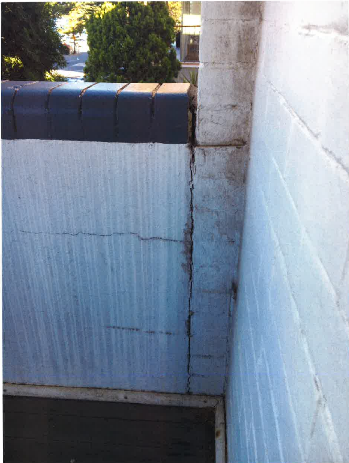
P13 – Separation of first floor balcony balustrade from façade brickwork.
