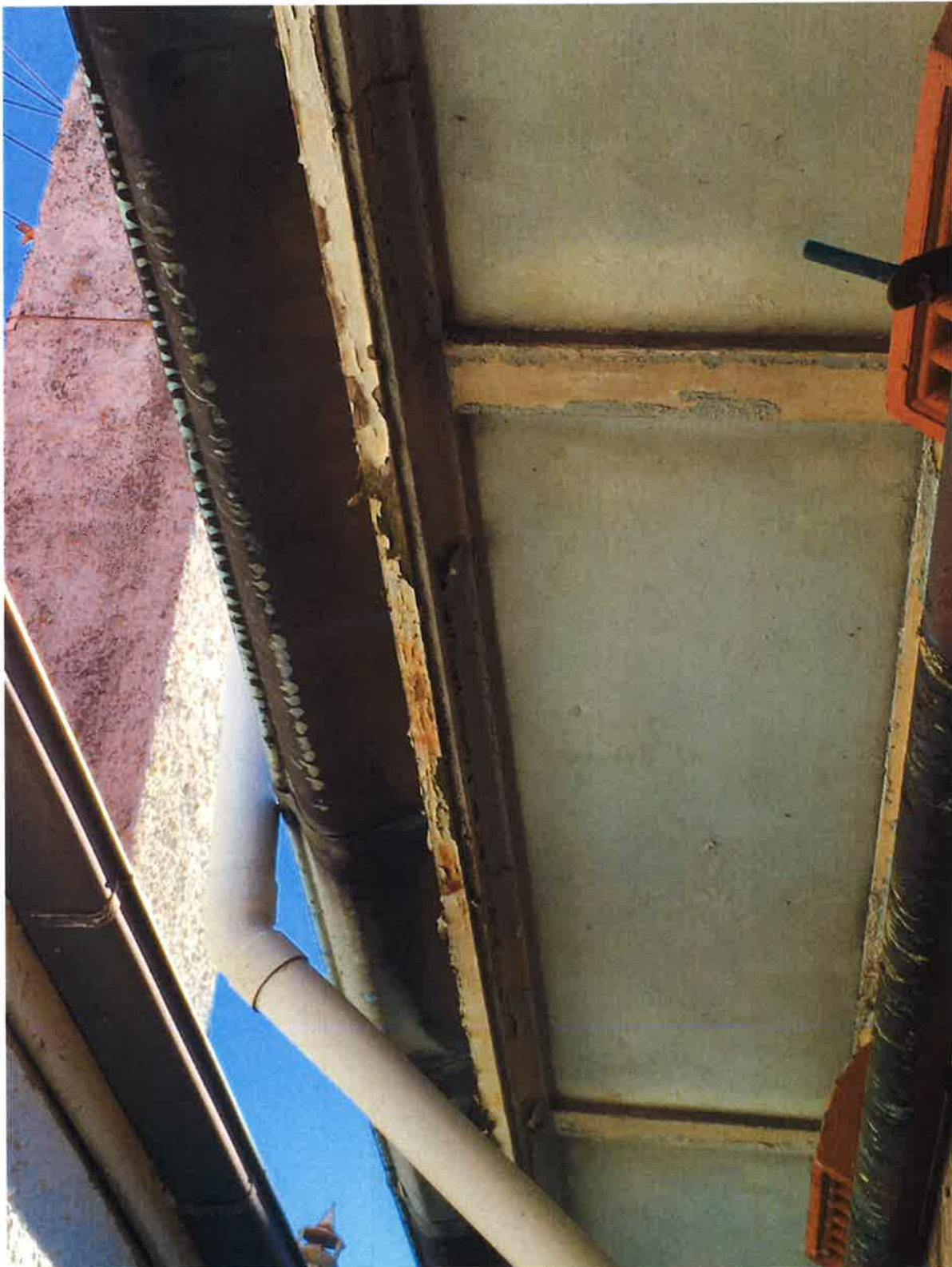
P19 – Detached eaves gutter to south-western side of building and asbestos eaves lining.
