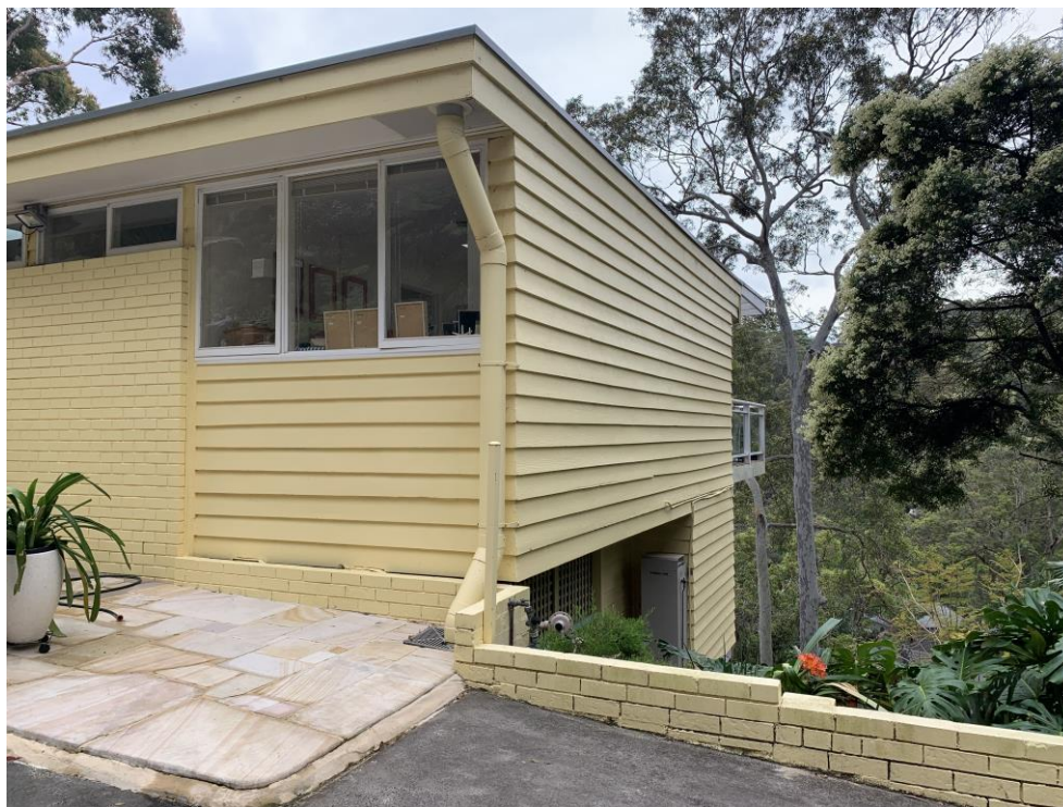
Fig 4: View looking north along existing eastern wall and the location of the new additions and garage
