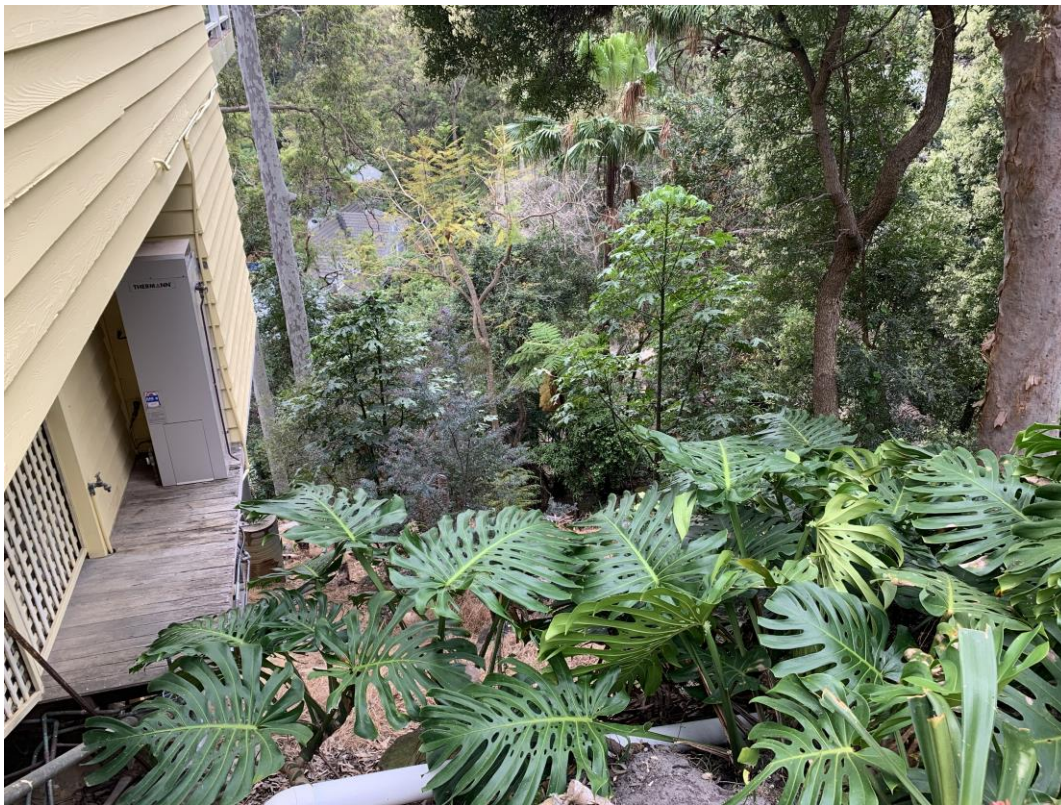
Fig 6: View looking north over the lower level of the dwelling and the location of the new additions
