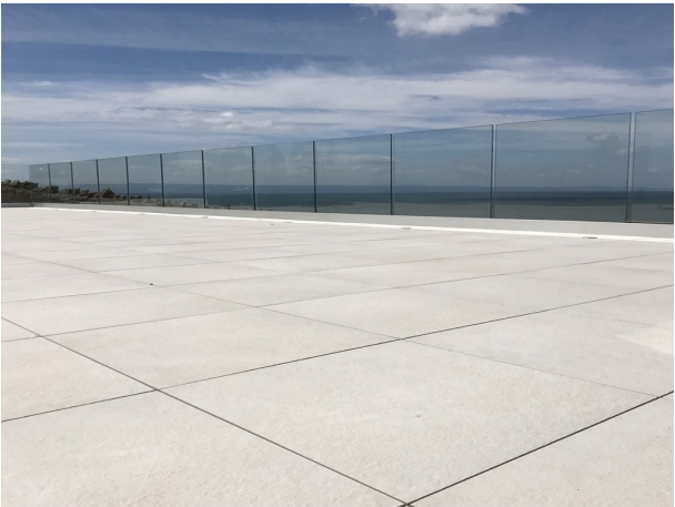
NATURAL STONE TILED DECKS
