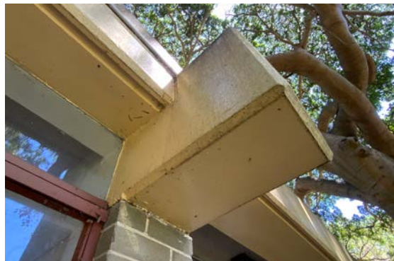
Figure 6: Detailed view of cementitious beam.
