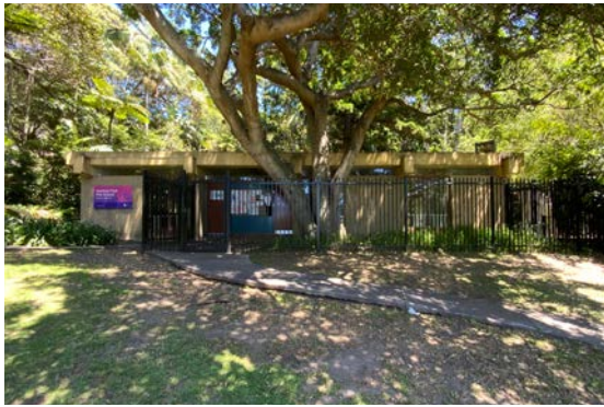
Figure 3: View of the entry elevation of the building.
