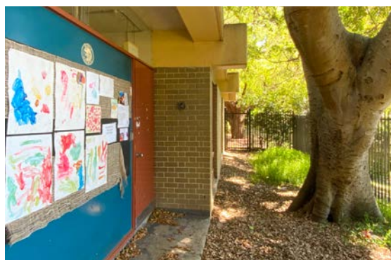
Figure 10: Detailed view of the eastern elevation.
