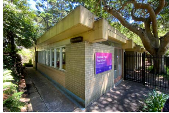
Figure 12: Detailed view of the cementitious roof beams and front elevation.
