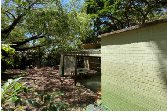
Figure 11: View of the western elevation and pergola.
