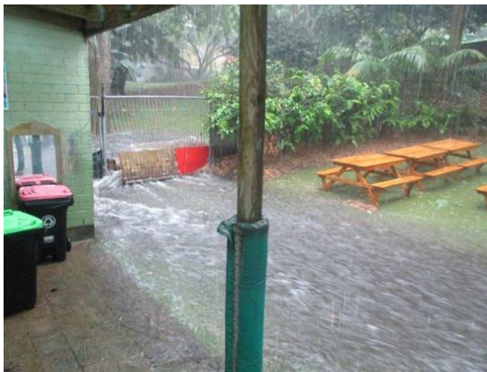
Figure 35: View of recent stormwater inundation across the children's play area.
