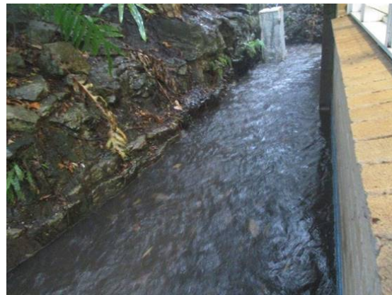
Figure 36: View of the southern elevation of the building showing significant flash-flooding around the perimeter of the building.
