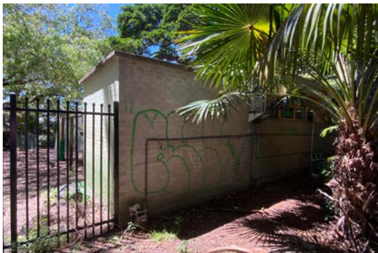
Figure 5: View of the rear of the site.
