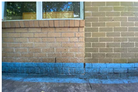
Figure 8: Detailed view of side elevation brick work.
