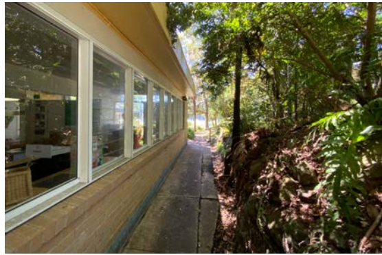
Figure 4: View of the southern elevation facing east.
