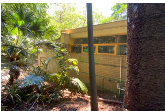
Figure 9: View of the southern elevation.
