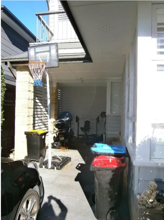
VIEW OF EXISTING SMALL CARPORT AND ENTRY AREA- THIS AREA TO BE ENCLOSED TO FORM A STUDY/GYM ROOM AND ENTRY TO BE RELOCATED.
