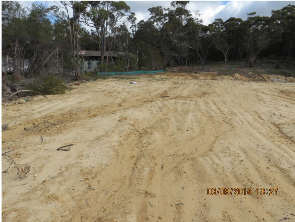
Figure 2.8. The development area has been cleared and graded to an even easterly aspect slope. The RFS building can be seen in the background.
