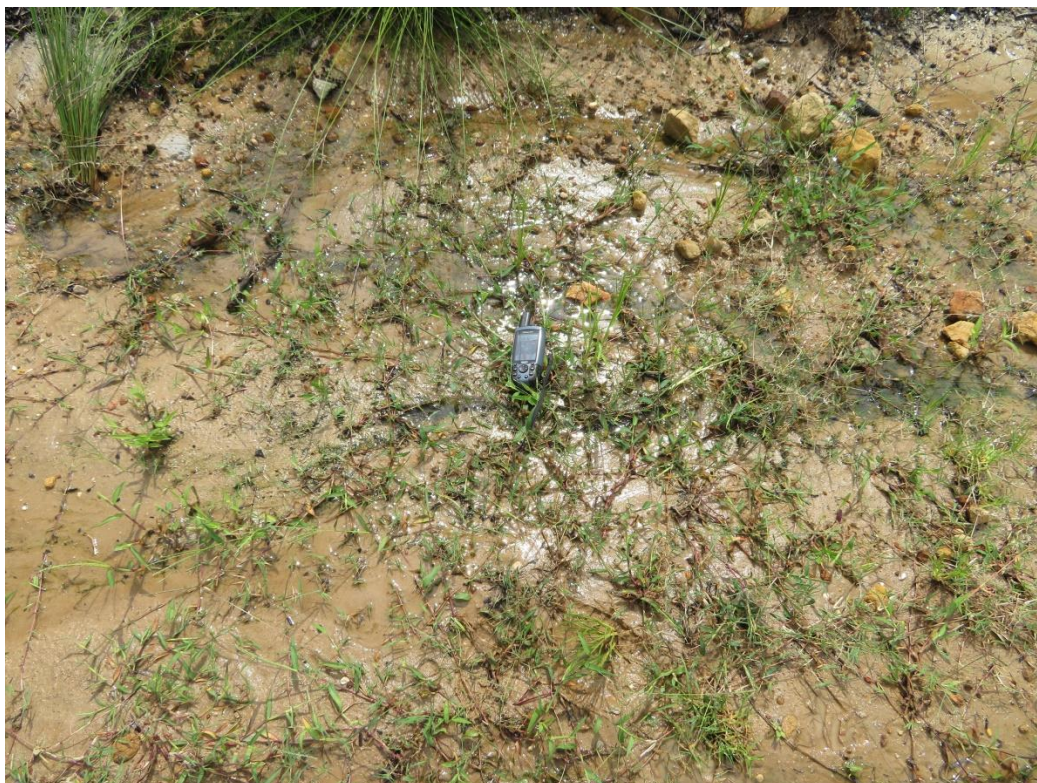
Figure 3.5. The stormwater runoff has created saturated sands in some areas during March 2017. Photo date 20.3.2017.
