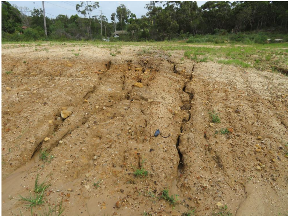
Figure 2.13. There is a bare slope near the northern border of the development area. This has been eroded since exposure in 2014. It needs to be turfed to prevent further loss of soil.
