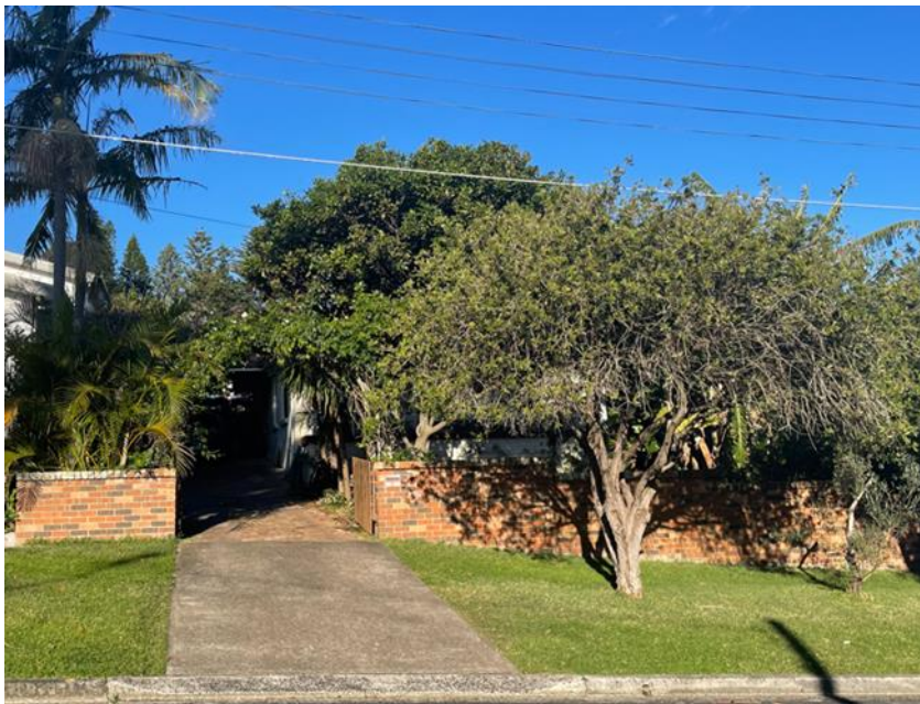
Figure 3 Existing street frontage of 3 Orana Road
