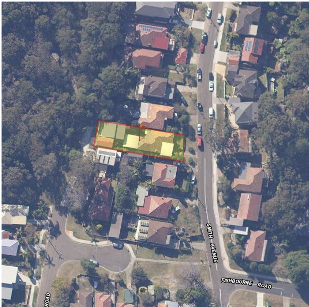
Figure 1: Site Location (Source: Six Maps)
