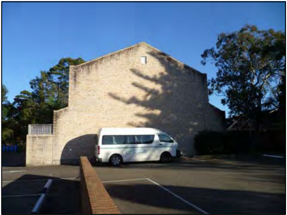
PHOTOGRAPH LOCATION 5 17-19 FORESTVILLE AVE
