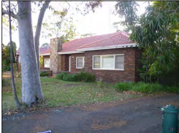
PHOTOGRAPH LOCATION 17 No.37 MELWOOD AVE
