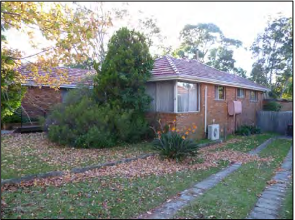
PHOTOGRAPH LOCATION 15 No.35 MELWOOD AVE
