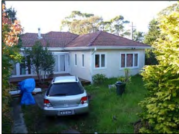
PHOTOGRAPH LOCATION 9 No.27 MELWOOD AVE
