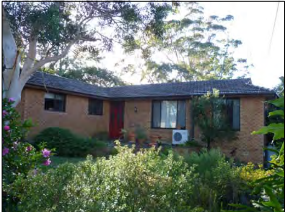
PHOTOGRAPH LOCATION 19 No.41 MELWOOD AVE
