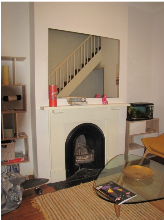
Figure 19: Original fireplace with cast iron insert and plan joinery surround – to be retained in front room.
