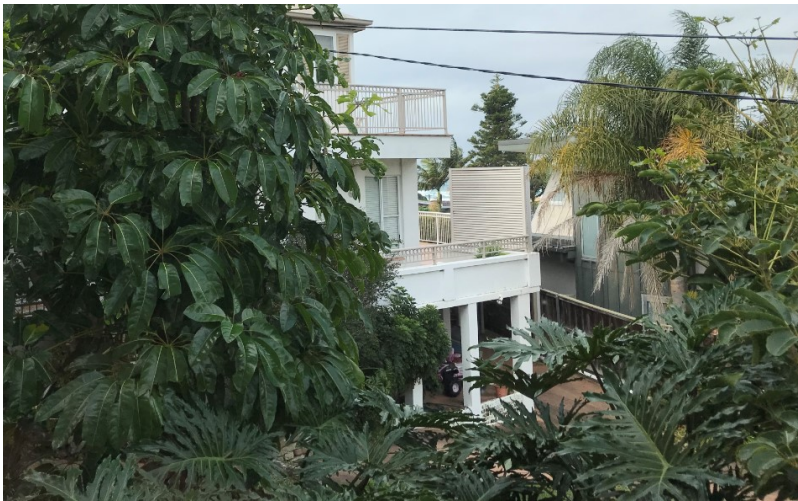
Figure 1: The Curl Curl beach views from No. 5 Bellevue Place, obstructed by unapproved privacy screen.
