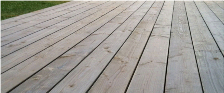
COVERED TIMBER DECKING Natural weathered grey hardwood decking; non-combustible bushfire resisting timber.
