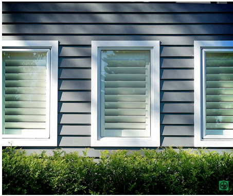
WINDOW TRIMS + ROOF FRAME: NON-COMBUSTIBLE TO COMPLY WITH BAL-40 Colour: White/Off Grey to match windows
