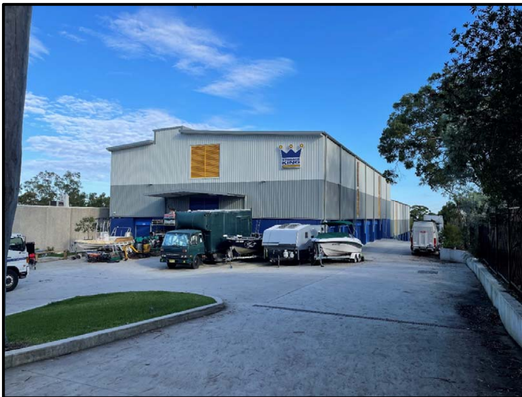
Photo 2 – View of Building 2, looking south east.
