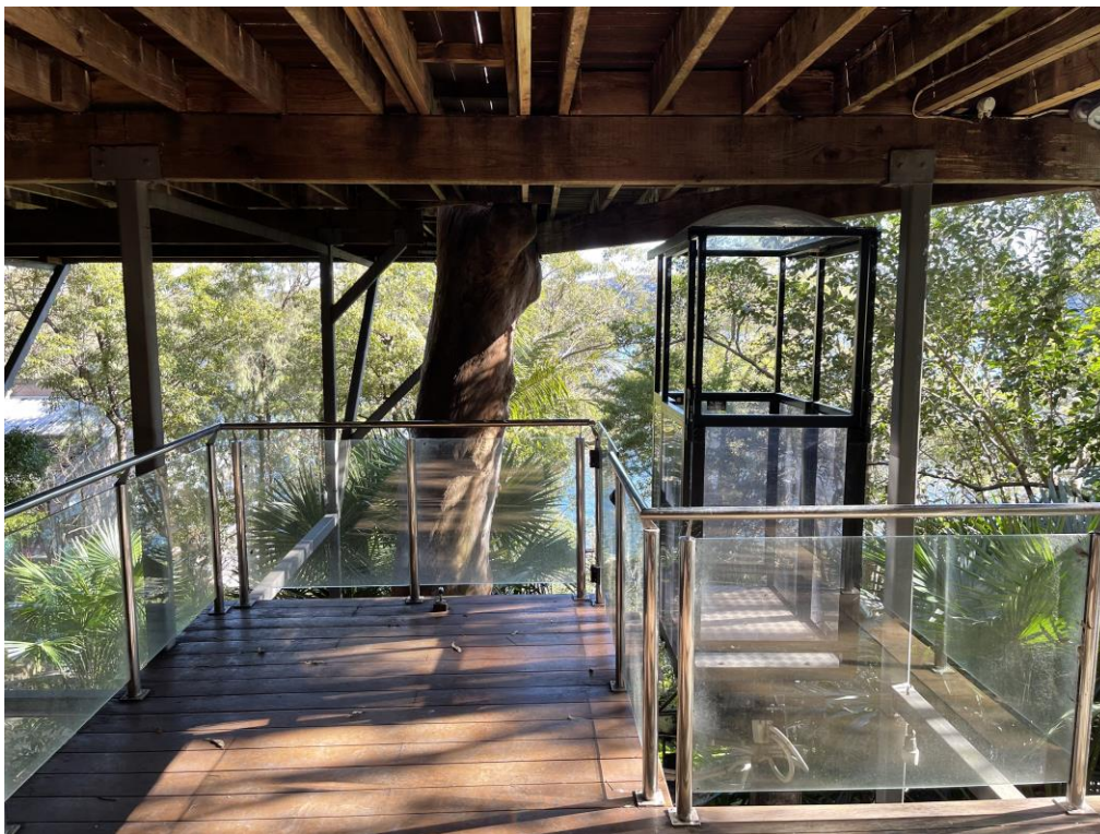
Fig 9: View of the existing building undercroft and inclinator station, looking west
