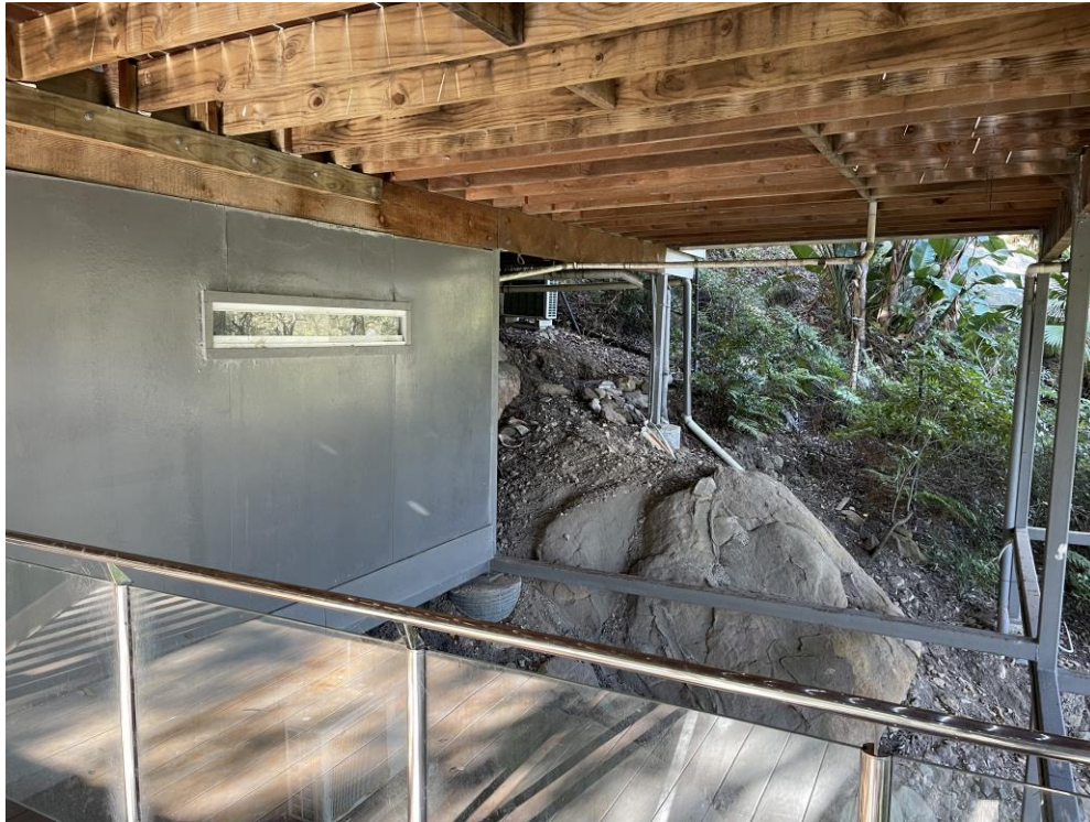
Fig 8: View of the existing building undercroft, looking south
