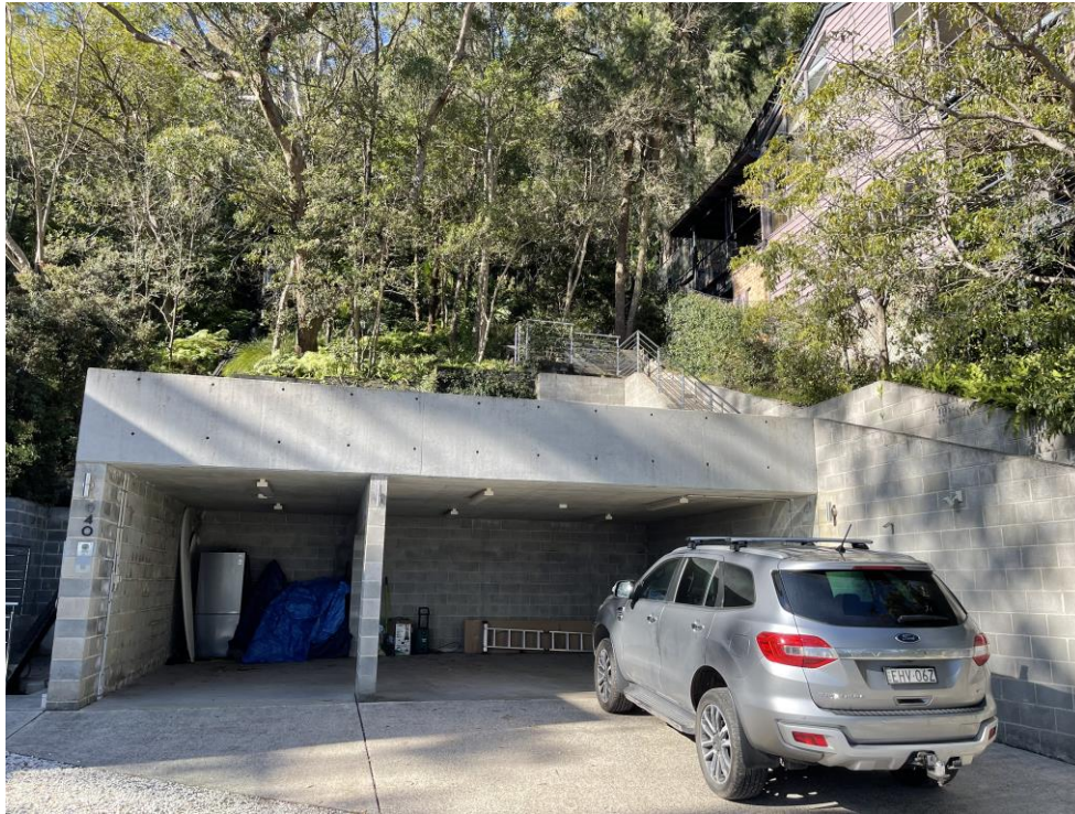
Fig 2: View of the site including existing garage, looking north-east from the common access driveway
