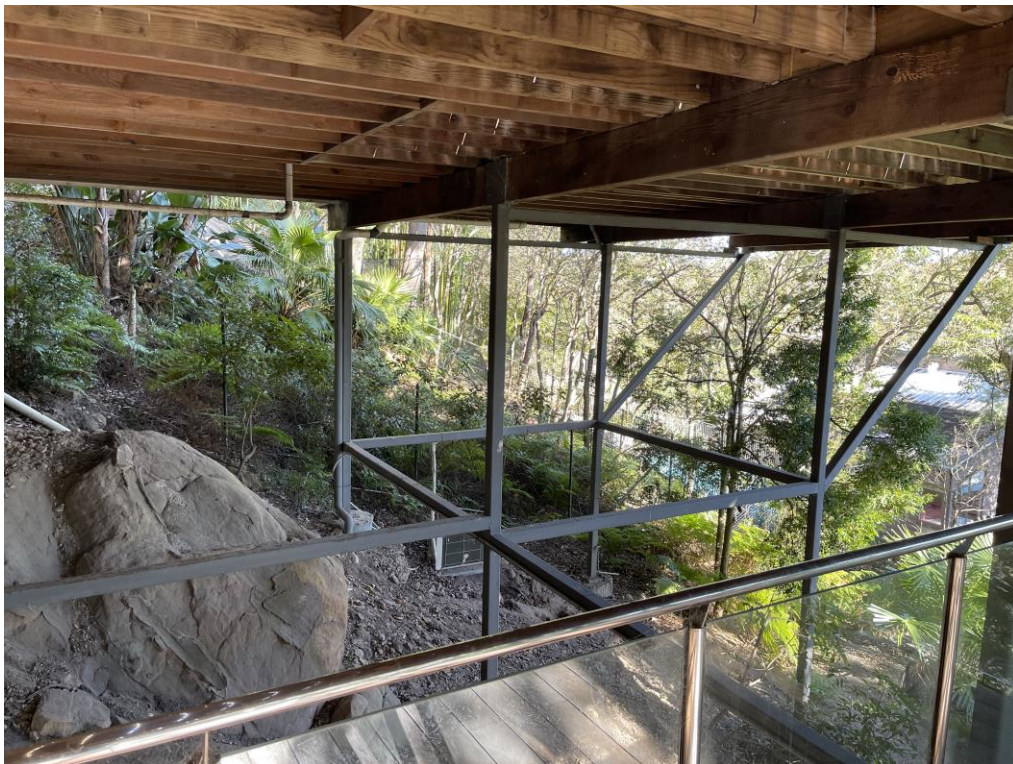
Fig 7: View of the existing building undercroft, looking south-west
