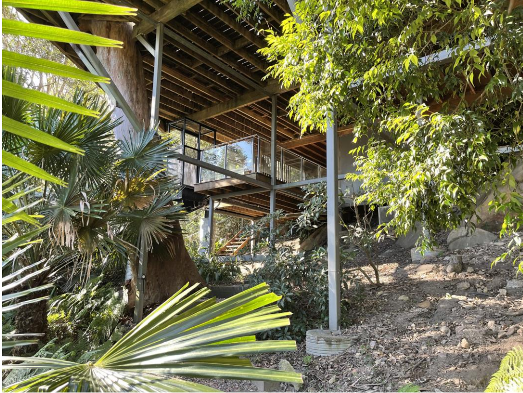
Fig 6: View of the existing building undercroft and inclinator station, looking north-east
