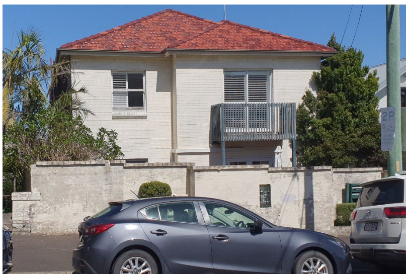
Fig 2 FRONT FENCE. Viewed from Ocean Road
