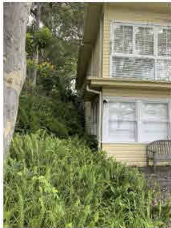
EXTG - REAR OF HOUSE
