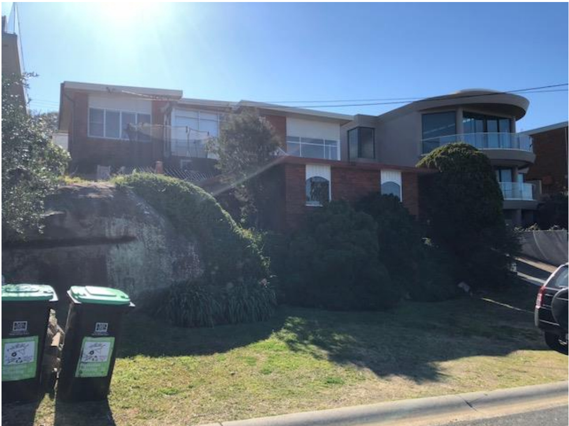
Figure 4. The existing single storey dwelling with garage in front
