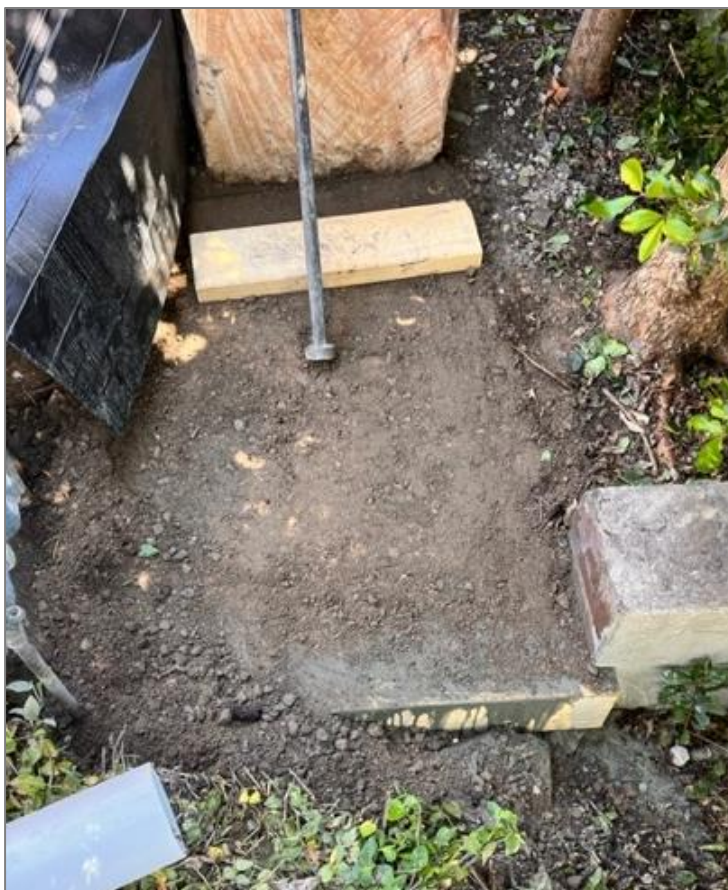
Plate 1 – Sandstone wall just completed near Group 3, note minimal footing construction.
