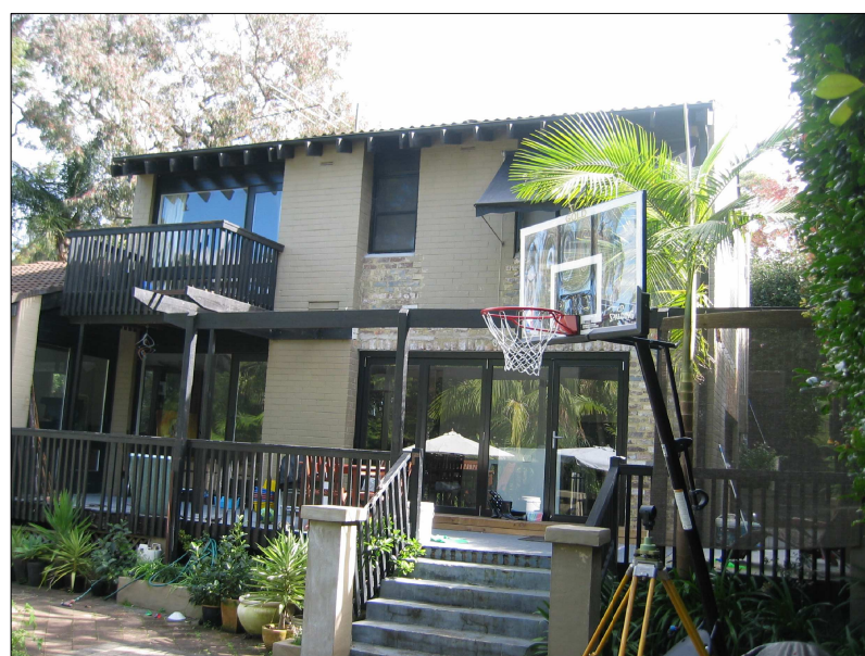
REAR ELEVATION LOOKING WEST
