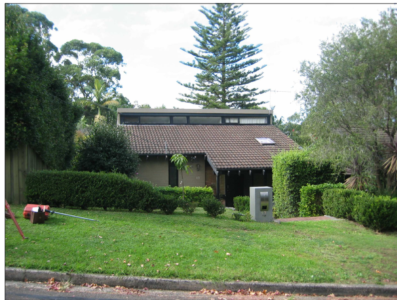
FRONT ELEVATION LOOKING EAST
