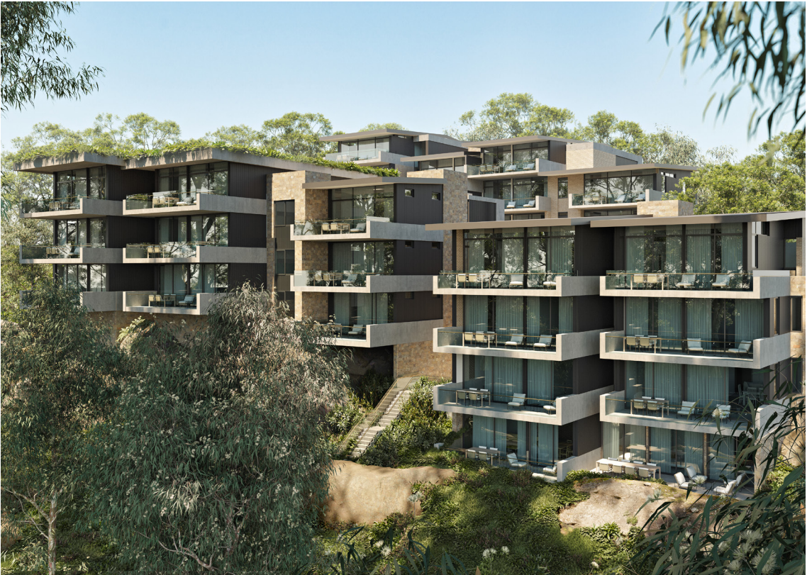
VIEW OF SITE FROM NORTH
