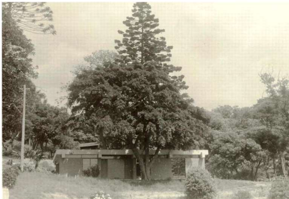
Figure 3: Ivanhoe Park Childcare Centre and Guide Hall 1964 (photo courtesy Northern Beaches Council Local Studies, Manly Library)
