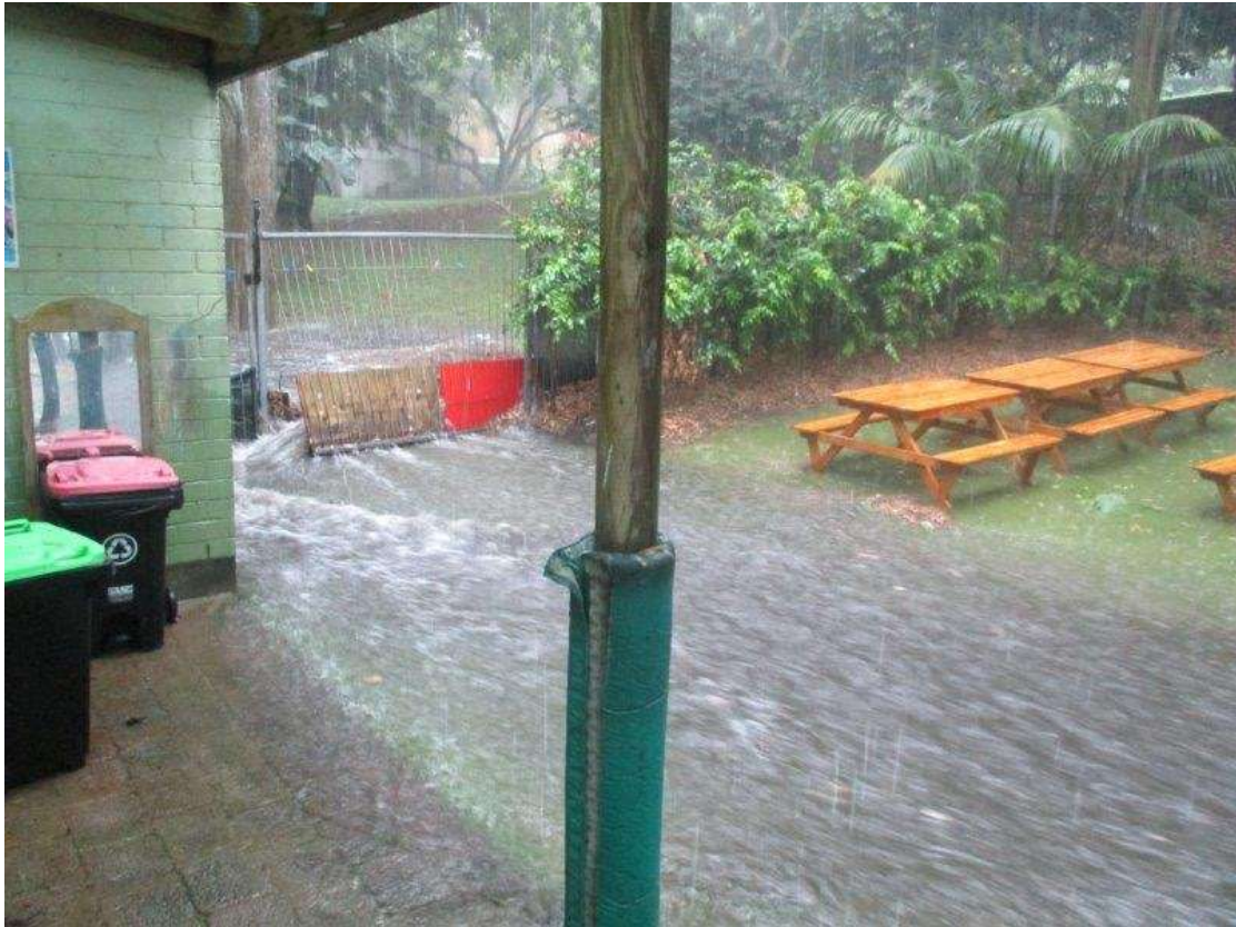
Figure 7: Flooding at the preschool November 2019
