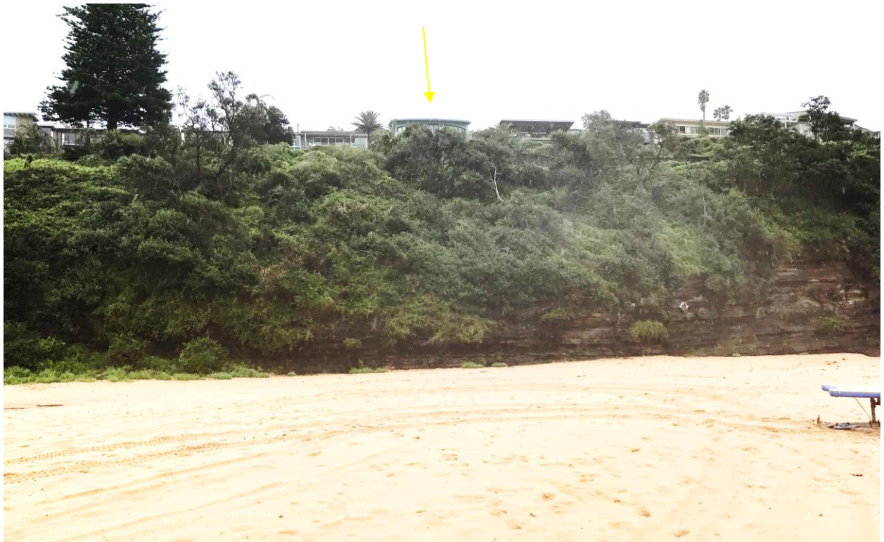
Figure 3: Broad view of cliff face SE of subject property (at arrow) on 25 February 2022, facing north
