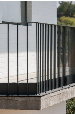
STEEL BALUSTRADE POWDERCOAT FINISH 'BLACK' OR SIMILAR WHERE MARKED ON ELEVATION.
